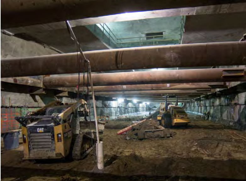
1 The station box is graded
