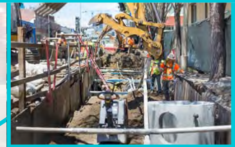
4th St. Surface Track, Systems (STS)
