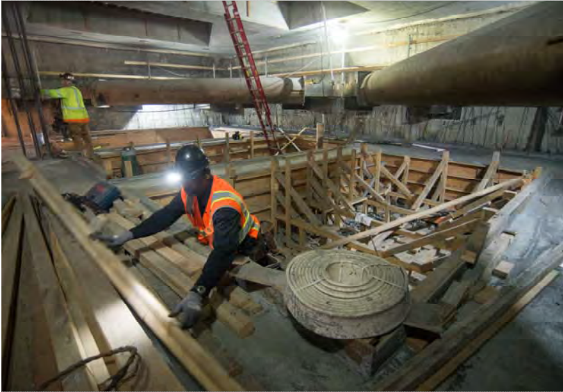
1 Workers remove concrete forms after pouring the floor slab
