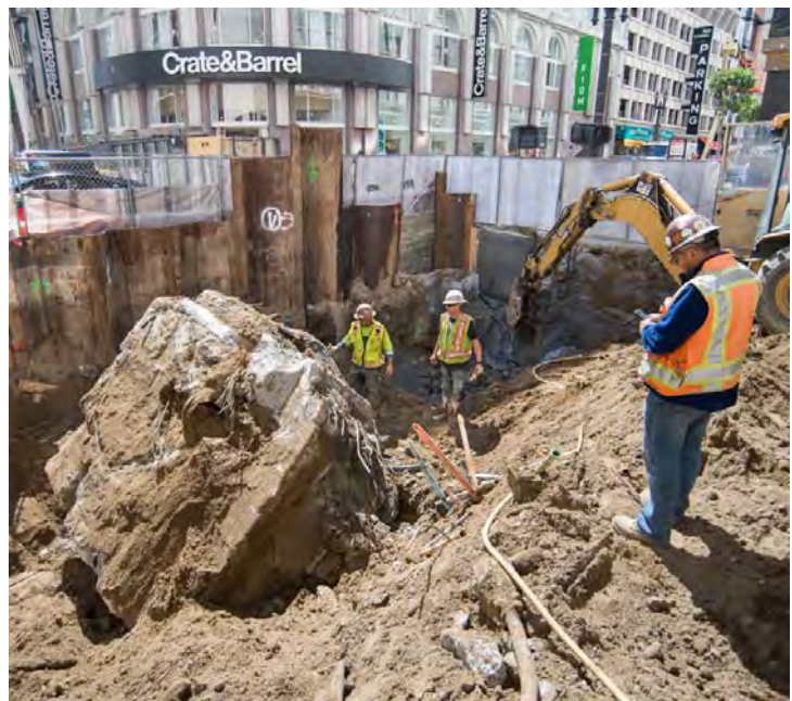
3 Obstructions are demolished and removed ahead of tangent pile work
