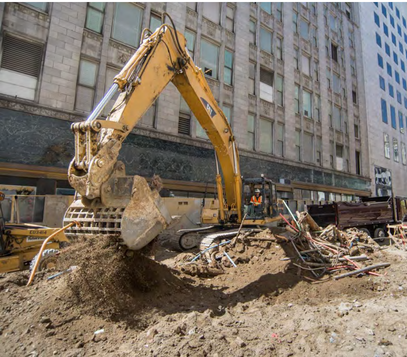
2 Material is excavated and old utilities are sifted and removed
