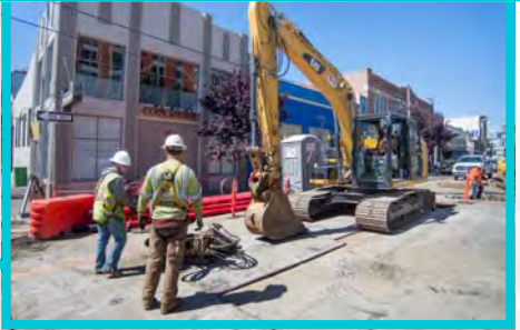
4th St. Surface Track, Systems (STS)
