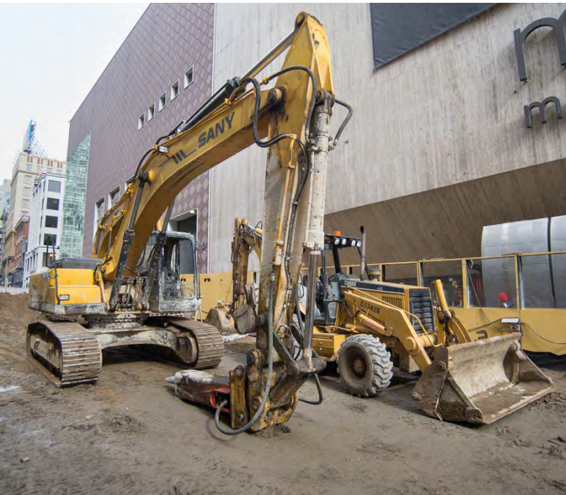
2 Heavy earth moving equipment is mobilized and support systems installed
