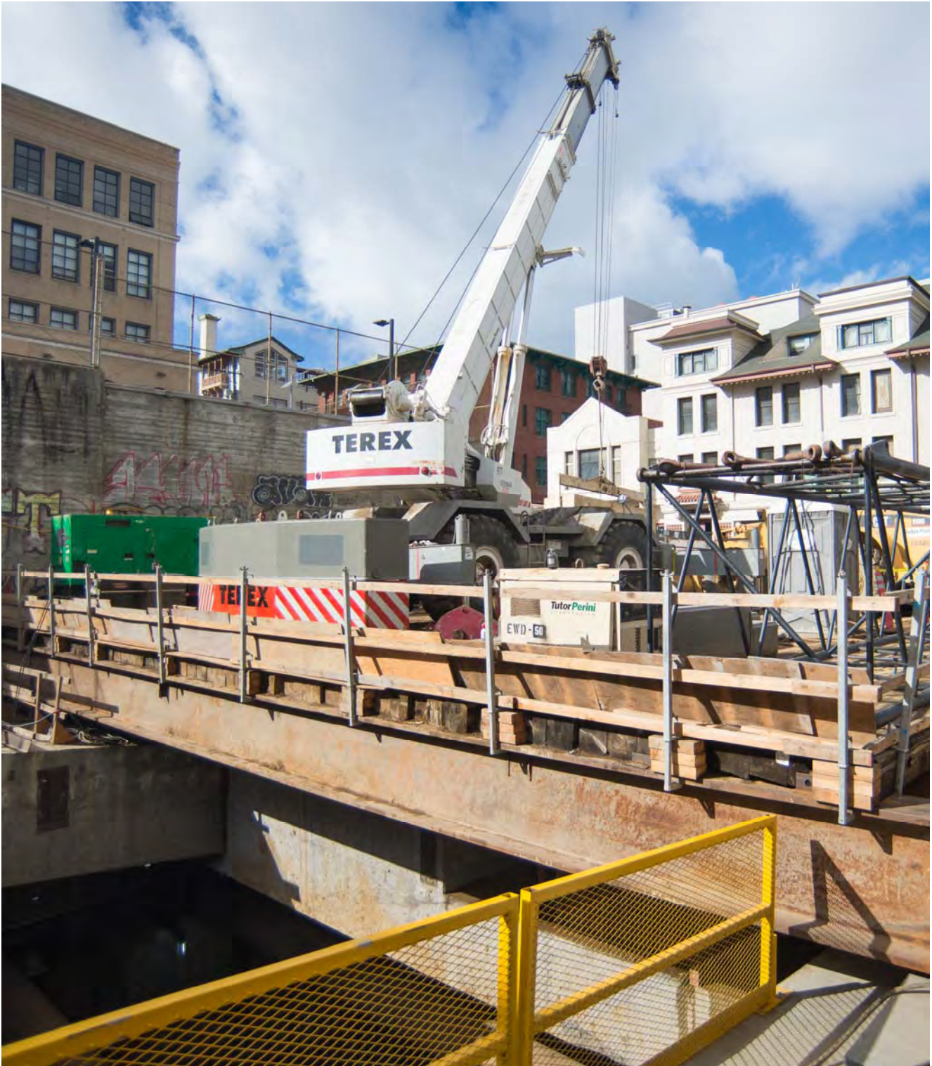
A large crane is used at the Chinatown Station site to lift excavated soil out of the headhouse for transport offsite.
