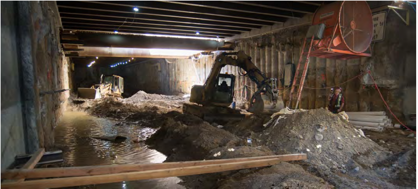
A mechanic inspects work on a ventilator fan inside the south concourse of the Union Square/Market Street Station, beneath the intersection of Ellis and Stockton.
