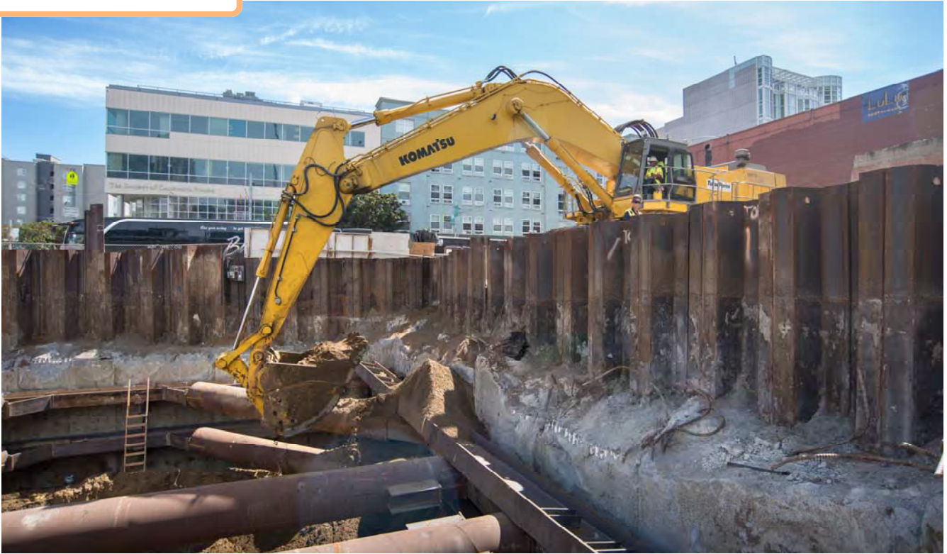
A large excavator removes material gathered from the station box interior.
