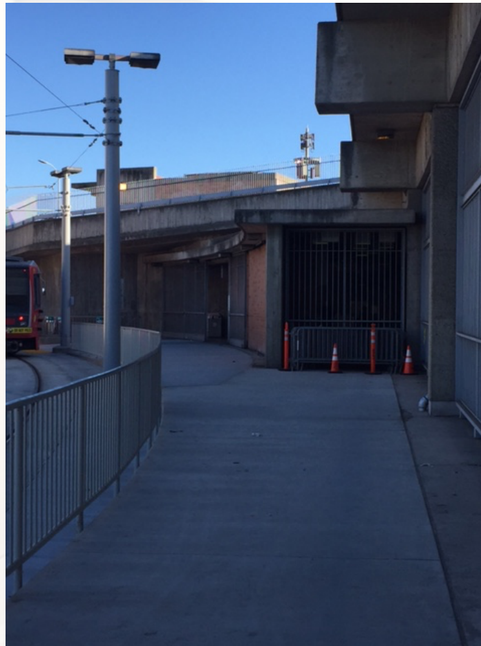
Concourse walkway to South Entry (free area) – Existing Conditions
