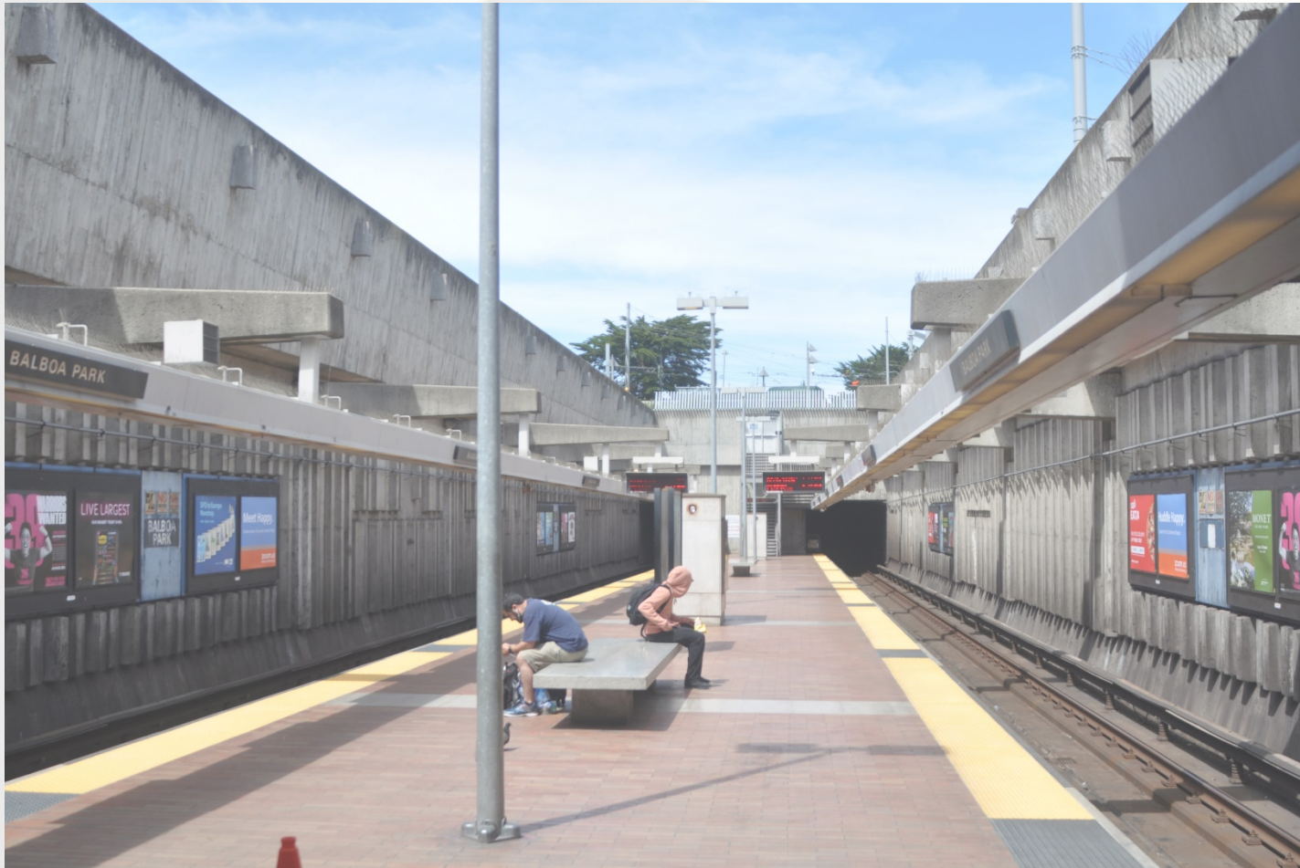
Platform Level (North end) – Existing Conditions
