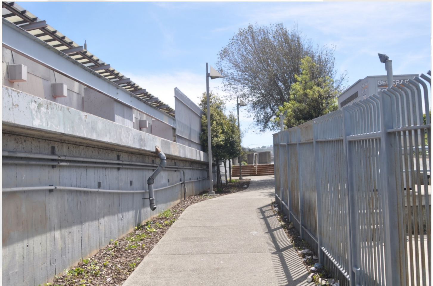
Westside pedestrian walkway (North to Geneva Ave) – Existing Condition
