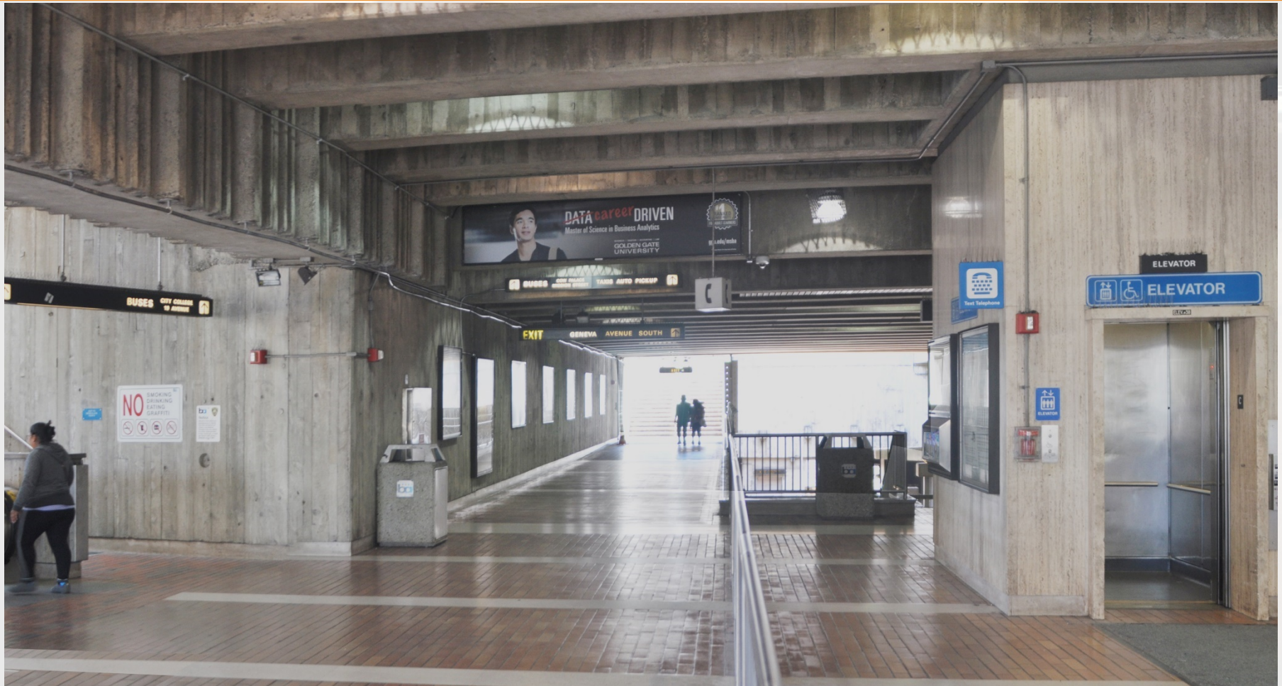
Concourse walkway to South Entry (free area) – Existing Conditions
