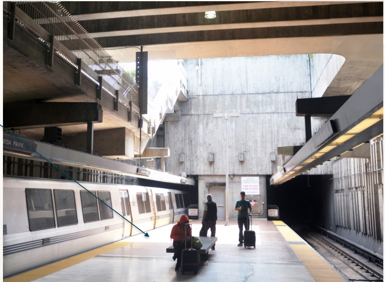
Platform Level (South end) – Existing Conditions
