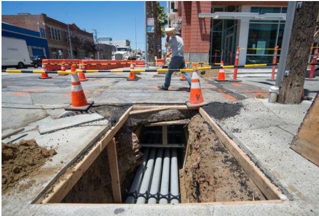
6. Surface, Track and Systems
