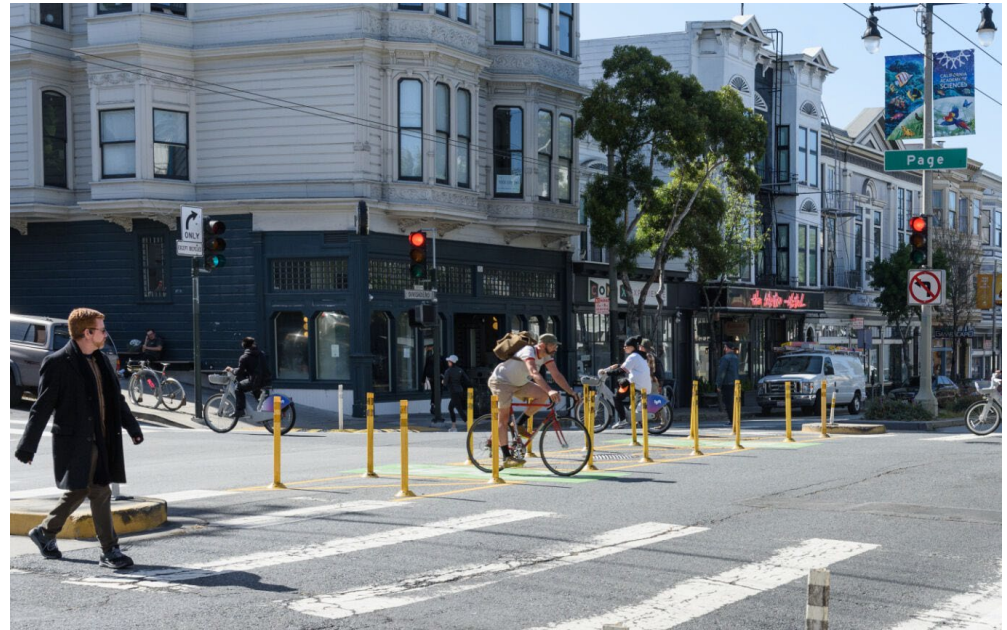
Diverter upgrades on Page Street (Page/Divisadero shown)
