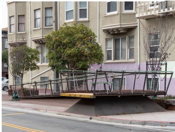
Accessible via Small Ramp
