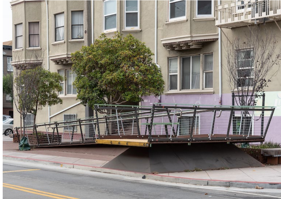
Example of “mini-high” ramp stop
