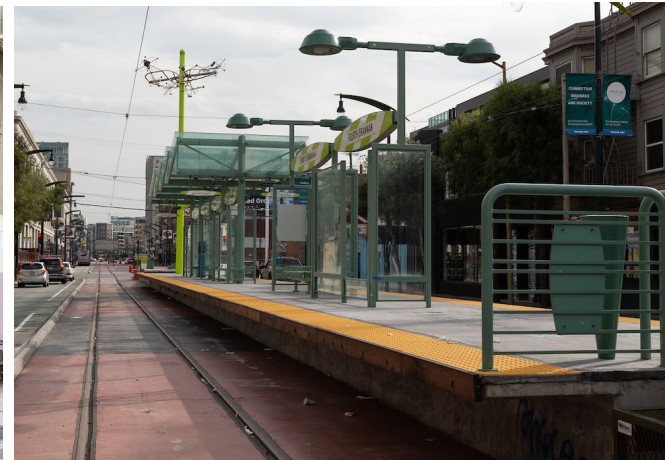
Full Level Boarding
