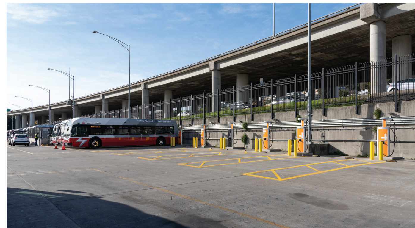
Figure 8-3: Charging Station at Woods Facility
