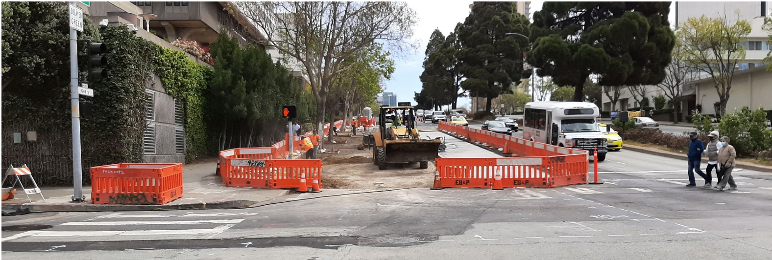
Example of bus bulb construction
