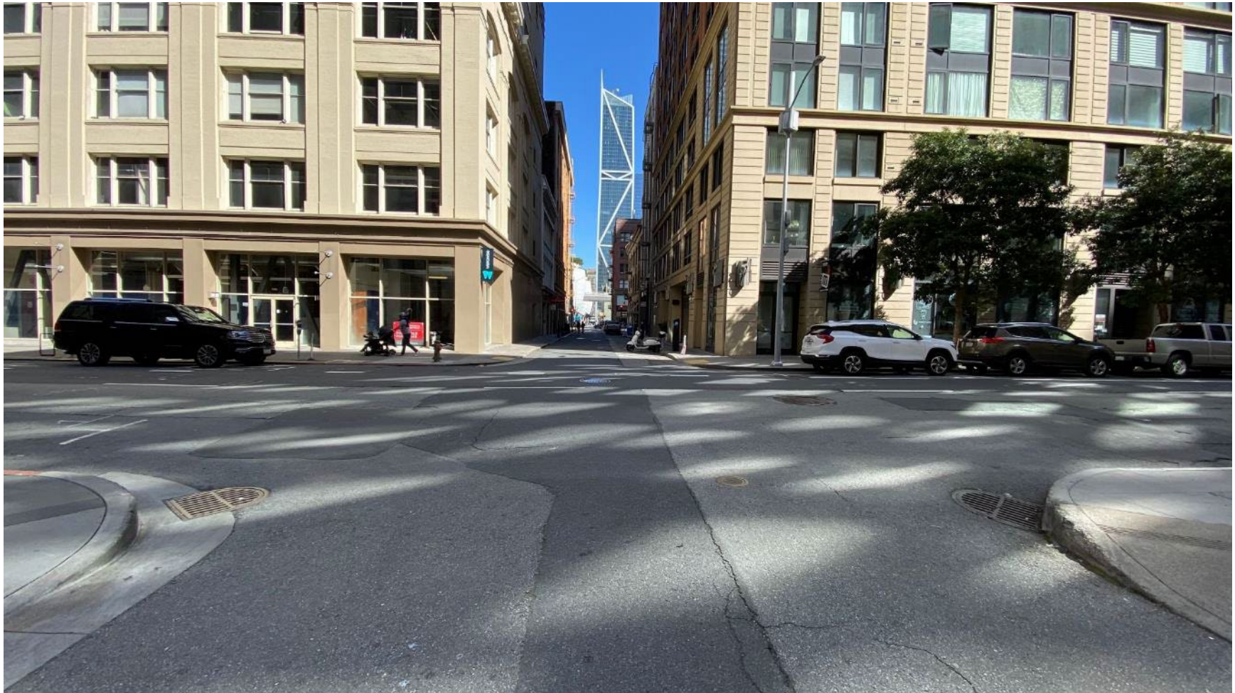
5 Natoma St. looking east toward New Montgomery St. - Traffic Signal and raised crosswalks proposed
