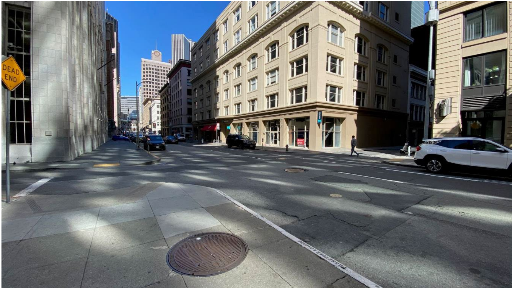
7 New Montgomery St. at Natoma St. looking northeast - Traffic Signal, raised crosswalks and bulbs (west/left side) proposed
