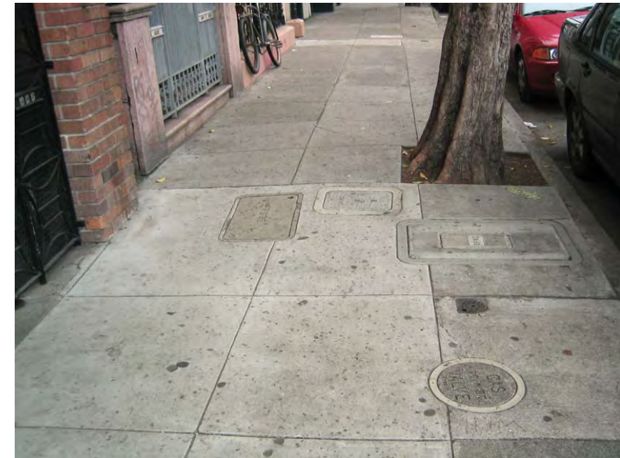
▲ Utilities are often scattered in the sidewalk without consideration for the overall streetscape environment
