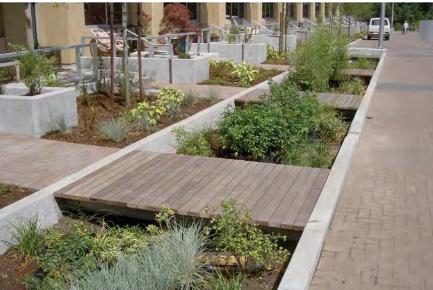
▲ This apartment building uses boardwalks over an infiltration area to define unique entrances to each unit from a shared public way Source: Sherwood Design Engineers
