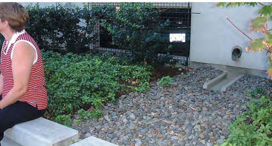
◀ Stormwater planters can be part of the building frontage zone, where roof runoff is temporarily detained, and used as an amenity to add greenery to the streetscape
