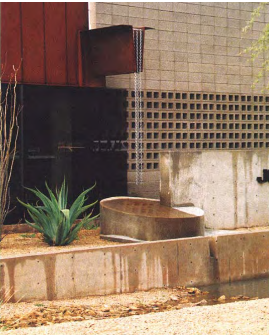
▲ This attractive architectural planter and fountain is a disconnected downspout that drains to a planter with an infiltration trench below
