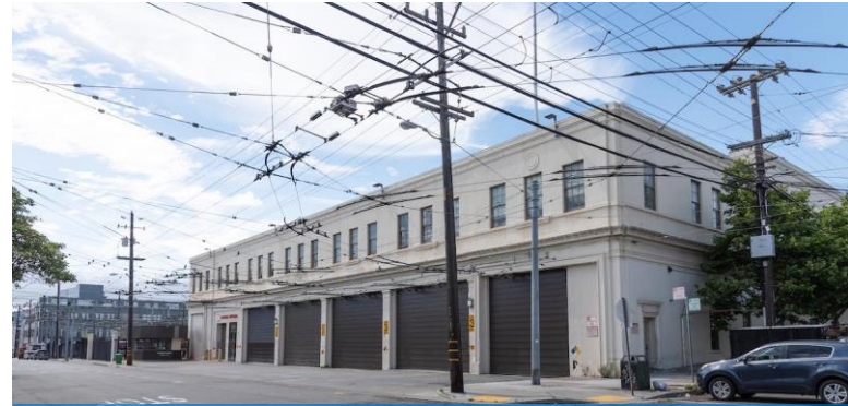
Seismic Upgrades & Building Replacement
