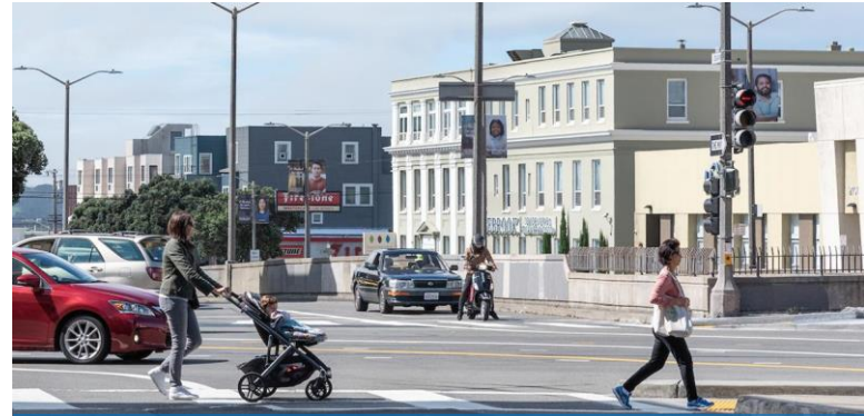
Corridor Pedestrian Safety Improvements
