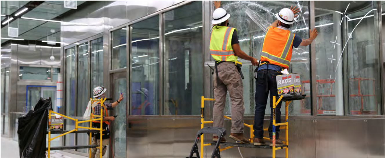
Workers putting anti graffiti film on the agent booth at UMS
