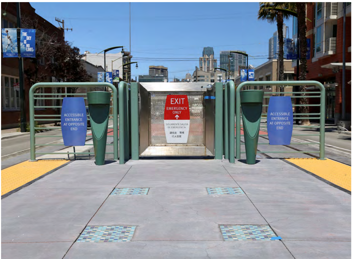
Exit signage at one of the STS surface stations
