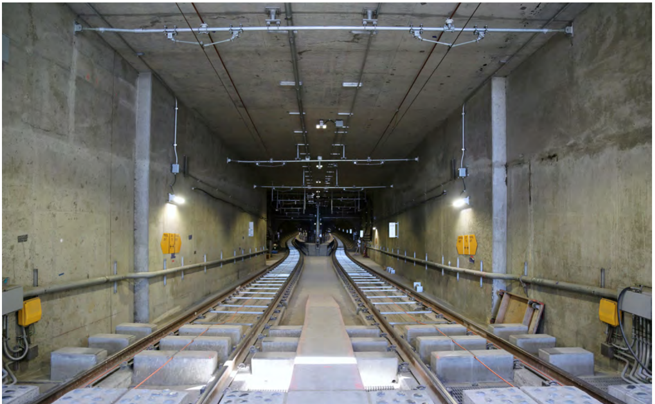
View down the Portal
