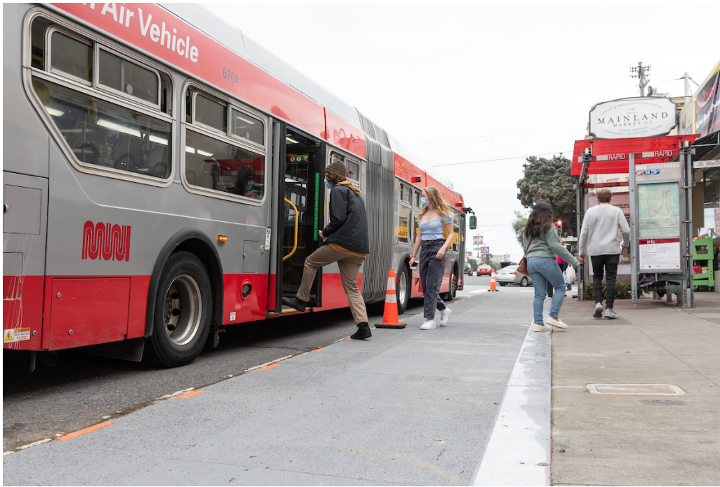
Figure 24: Temporary wooden bus bulb on Geary at 20th Avenue inbound bus stop
