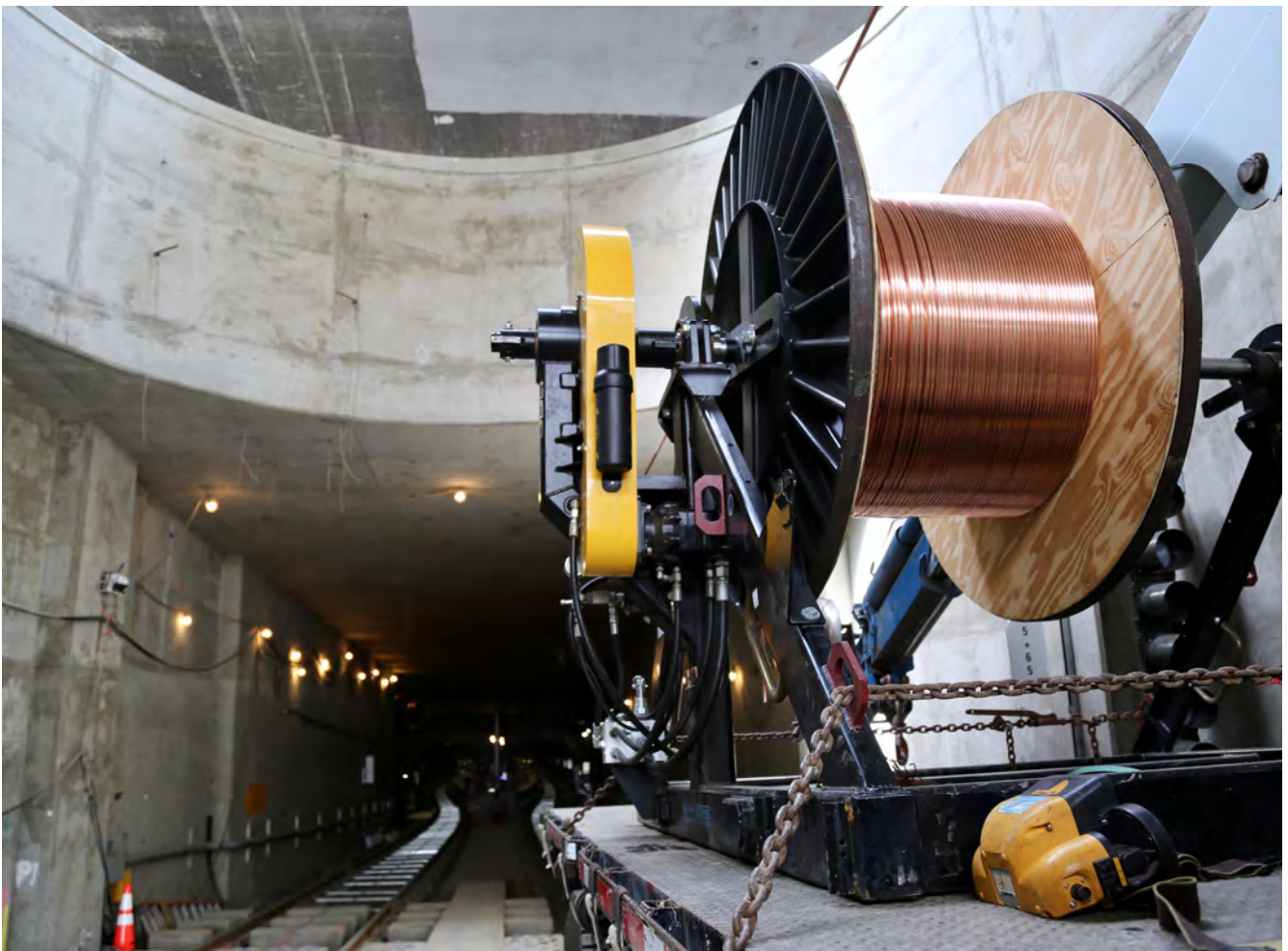
Contact line being pulled at the portal
