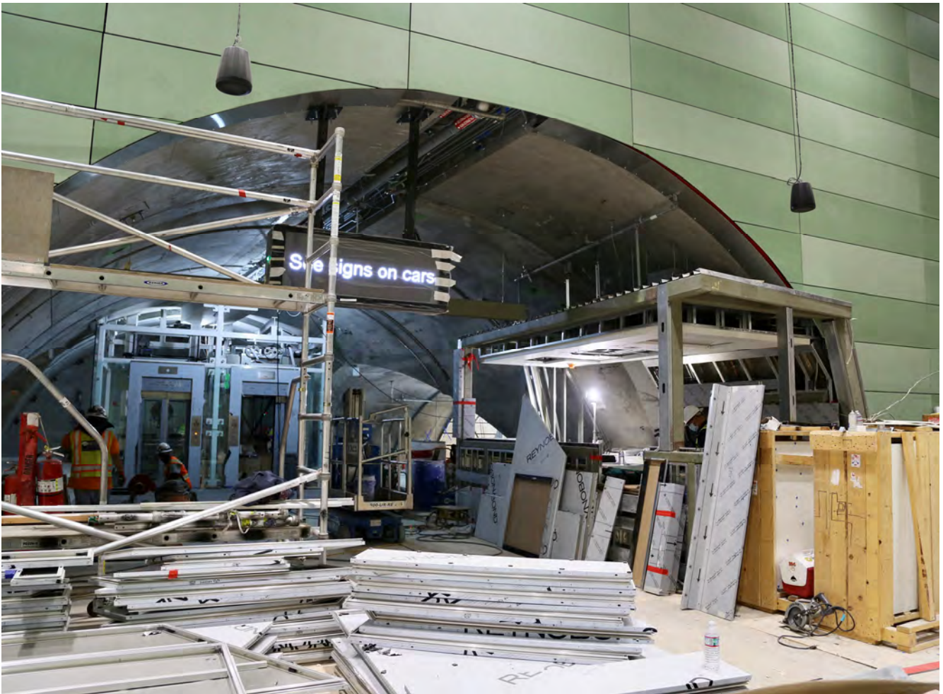
Panels ready to be installed at CTS
