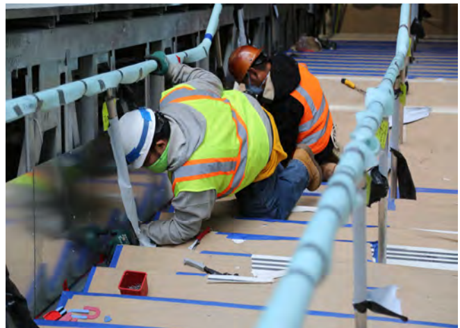
Workers installing the side paneling on the escalators.
