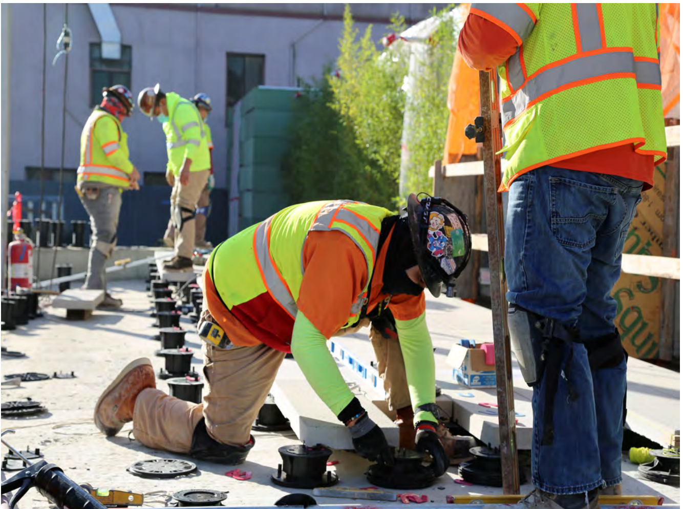
Workers installing the tile panels at China town station
