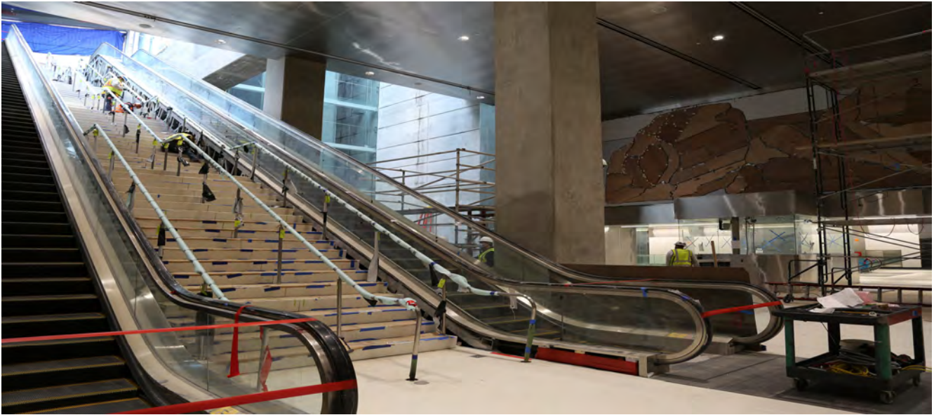
View of the escalator heading down to the ticketing hall at YBM
