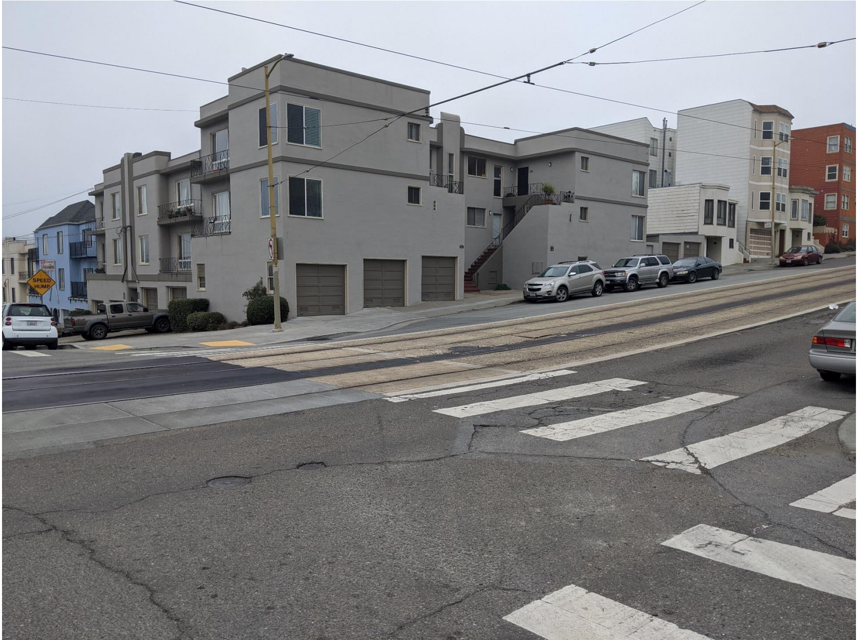
17 th St., approaching Judah St. – looking east
