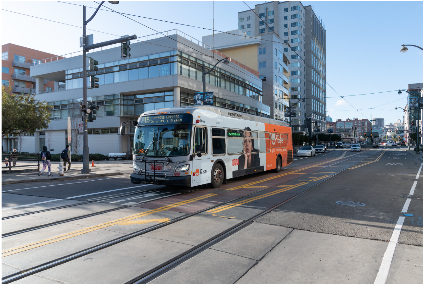
4th Street Bridge Temporary Emergency Transit Lanes
