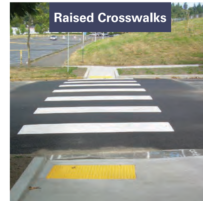
Raised crosswalks provide a level pedestrian path of travel from curb to curb. Vehicles are required to slow down before passing over the crosswalk, which is level to the sidewalk.
