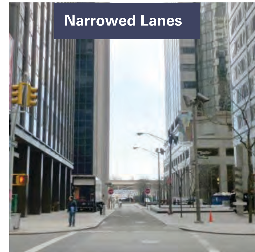
Narrowing lanes reduces existing lane widths. Lane narrowing can help reduce vehicle speeds and crossing distances for pedestrians.
