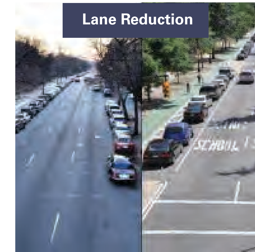
Lane reductions reallocate space from vehicles to people walking and biking. Reducing lanes is especially useful when there is excess capacity for cars.
