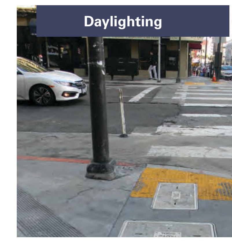
Daylighting is a cost-effective and quick way to increase pedestrian visibility by prohibiting parking up to 20 feet from the intersection.
