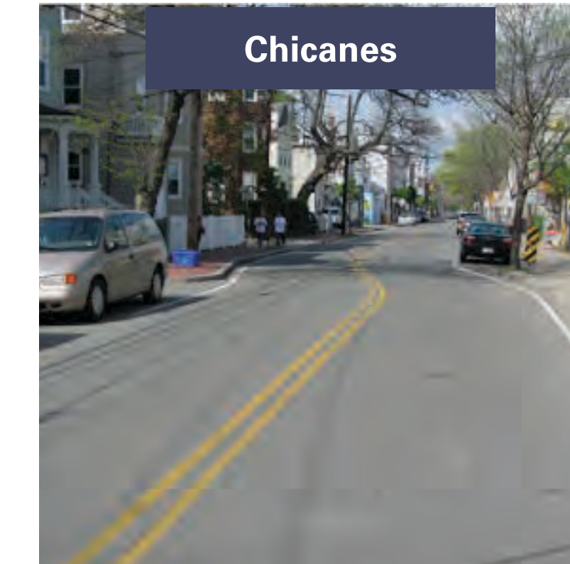
A chicane consists of offset curb extensions which help to narrow the roadway and reduce traffic speeds.
