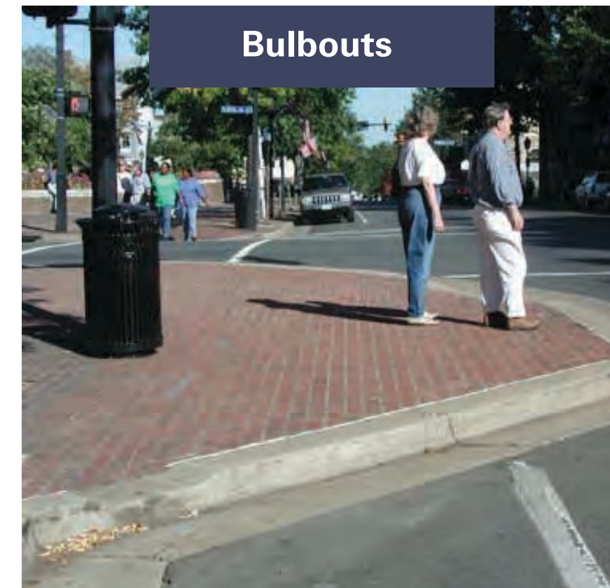
Bulbouts are extensions of the curb that visually and physically narrow the roadway to increase visibility of pedestrians and shorten crossing distances.
