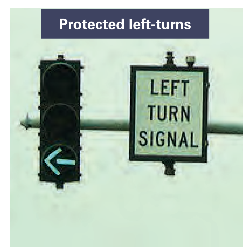
Protected left turns allow pedestrians to cross without driver conflicts by giving turning drivers their own dedicated phase for turns.
