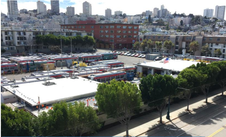
Kirkland Yard New Roof Layer & Drains
