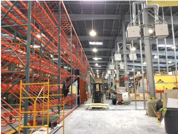
Burke Reconstruction Project
