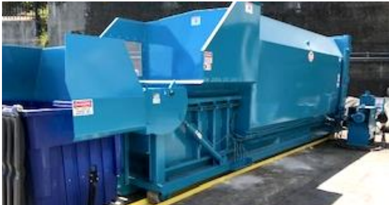
Woods Yard New Trash Compactor
