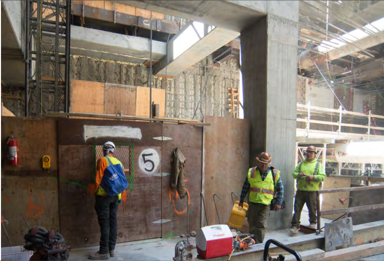
Workers have finished most major floor slabs and reinforced concrete walls
