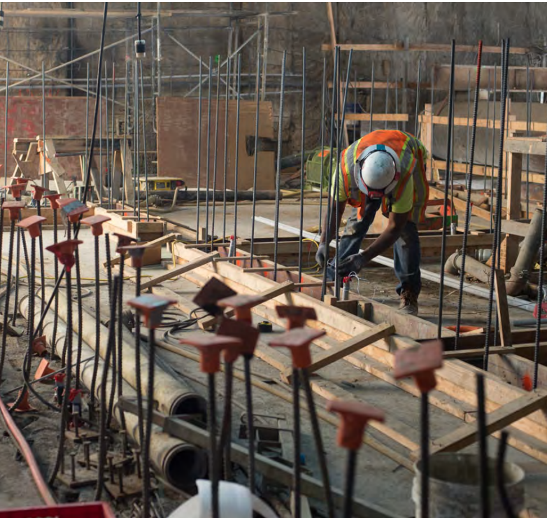
Crews continue building out interior walls by building forms for footings
