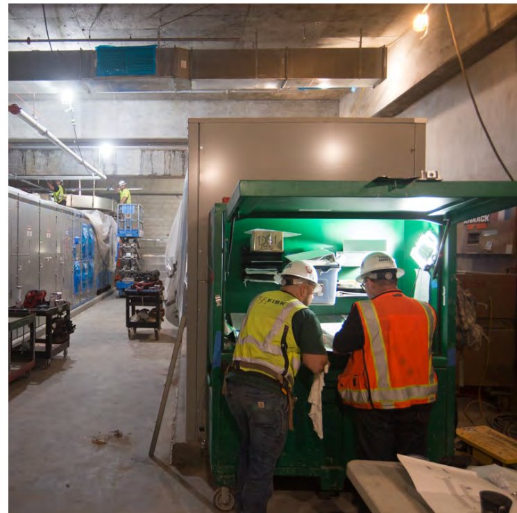
Electrical, ventilation, and signaling systems are being installed
