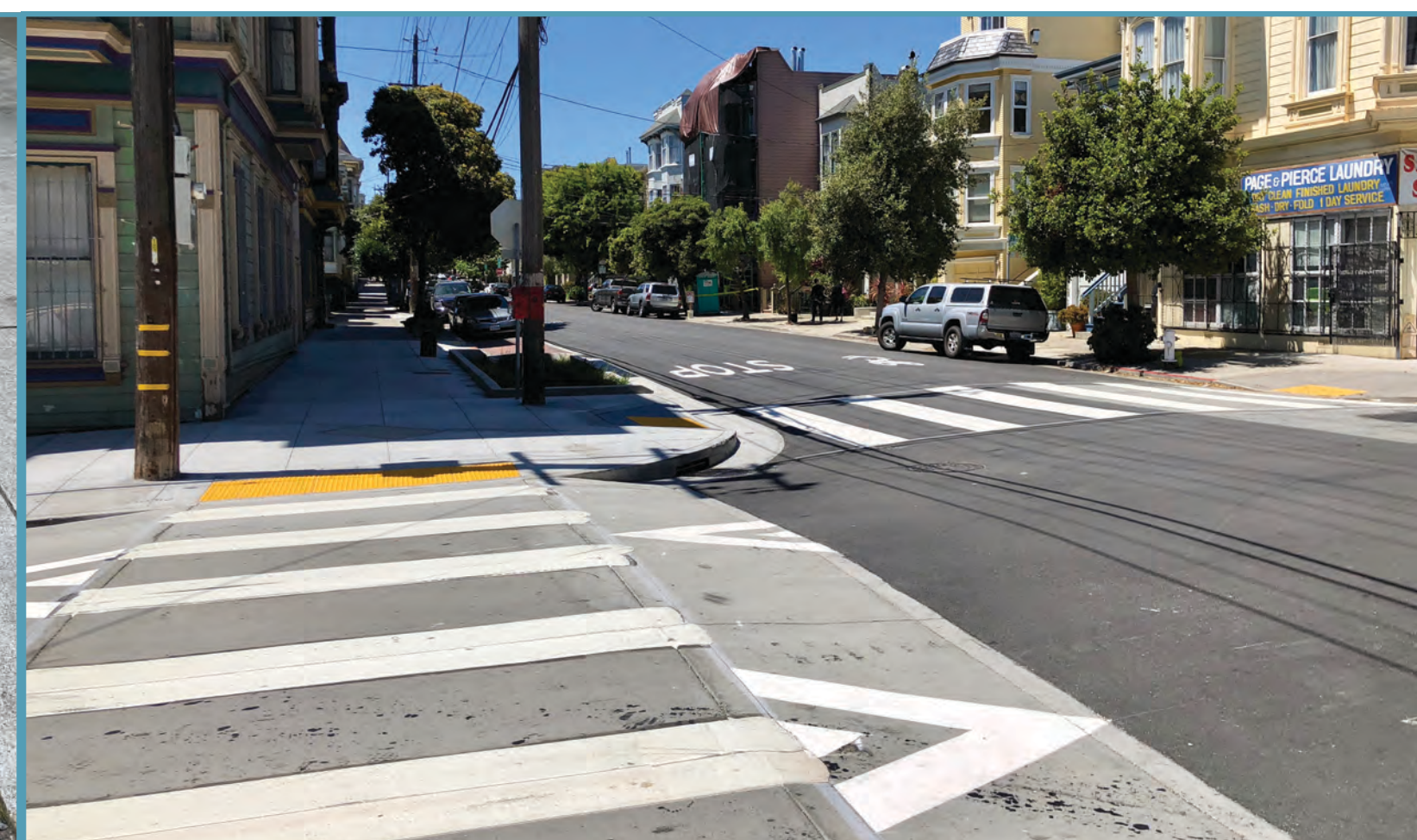
Raised crosswalks slow traffic and could be used at the Fell and Gough entries to Patricia's Green.
