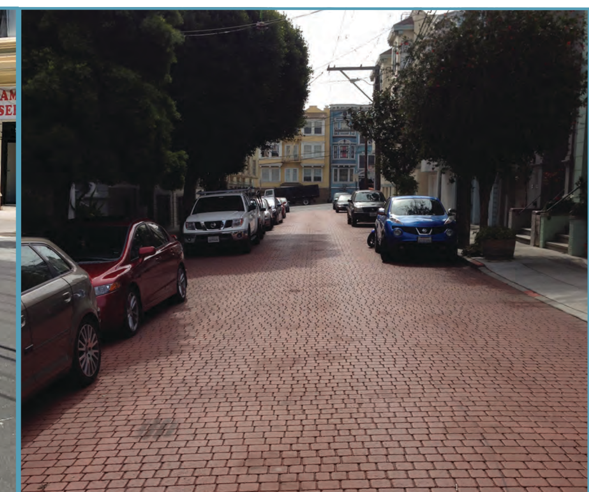
Stamped/colored asphalt calms traffic and creates a more neighborhood feel.
