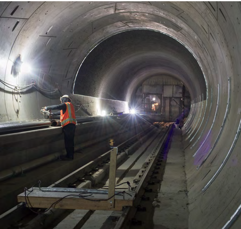
2 Concrete is poured, walkways are added, and utility brackets are installed
