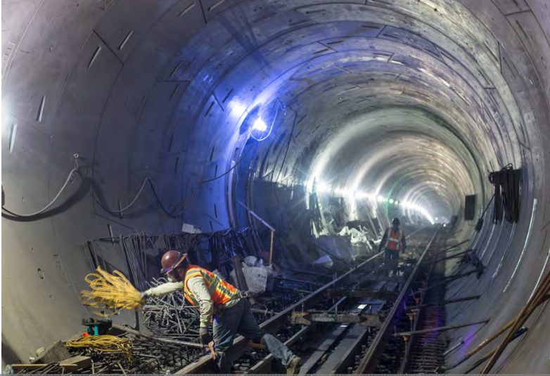
1. Workers install rebar and rails atop a steel framework
