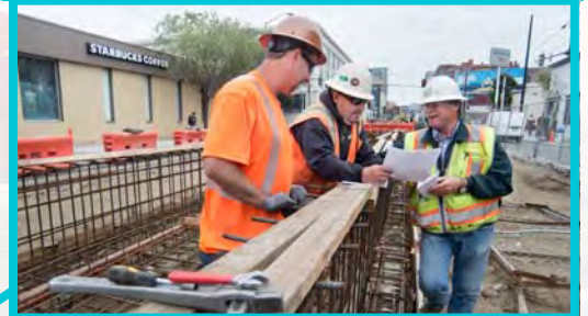
4th St. Surface Track, Systems (STS)
