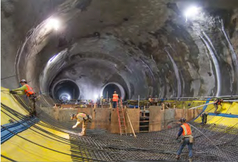
1. Crews install waterproofing against the outer walls of the cavern shell
