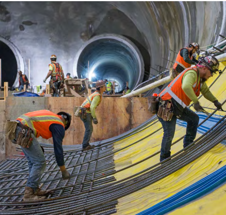
2 Rebar cages are constructed atop the waterproofing
