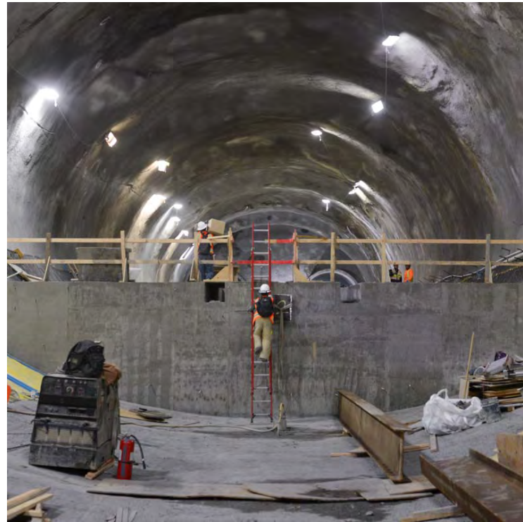
3 Crews pour concrete and remove the formwork as they go
