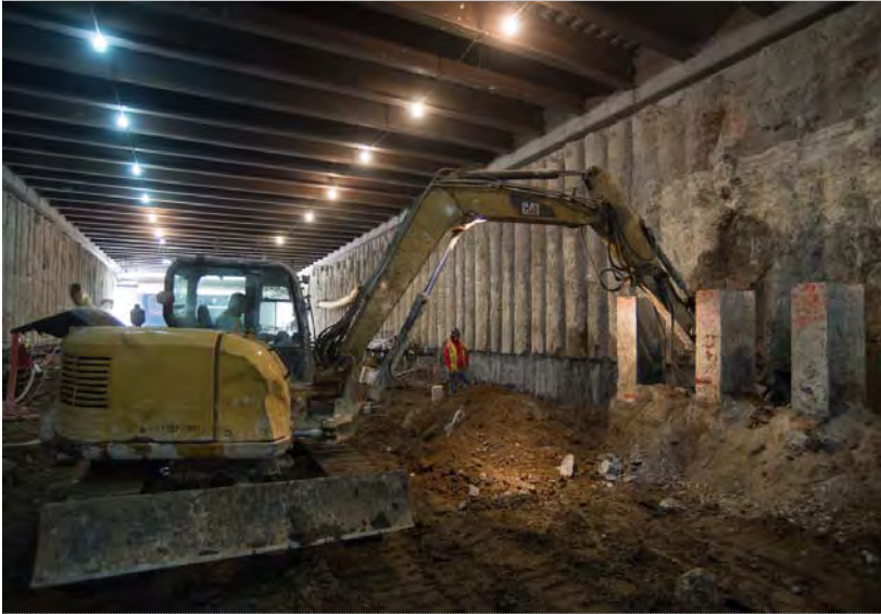
1 Excess concrete is removed and walls are prepared for steel brackets
