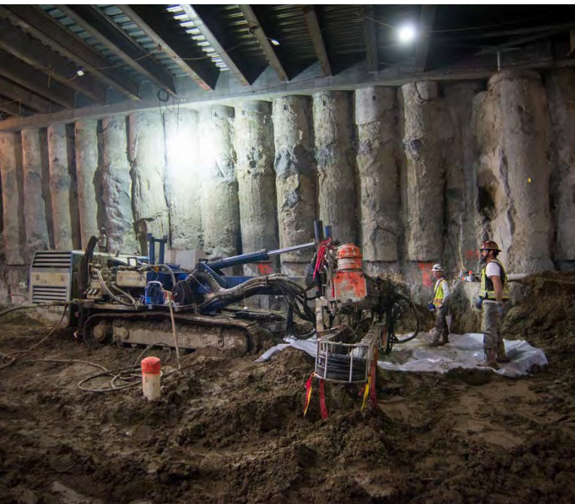
2 Compensation grouting work is performed ahead of bracket installation
