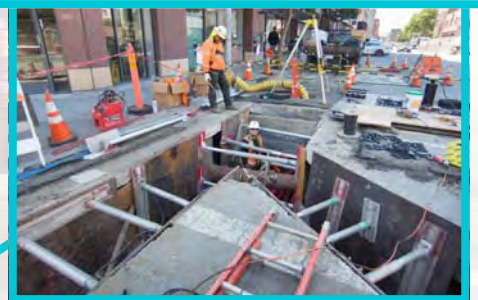
4th St. Surface Track, Systems (STS)
