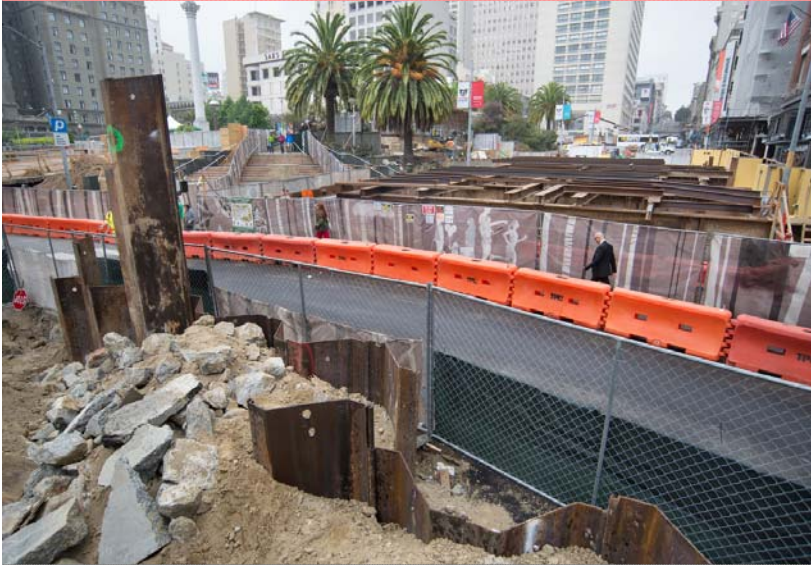
1 Traffic lanes are shifted over and steel sheet piles are installed
