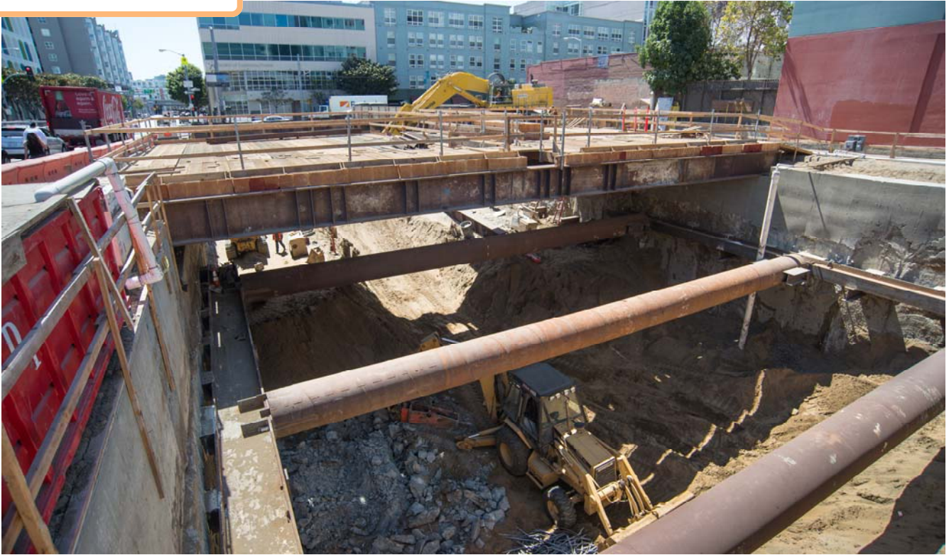
Steel supports called “walers” are temporarily installed during headhouse excavation.
