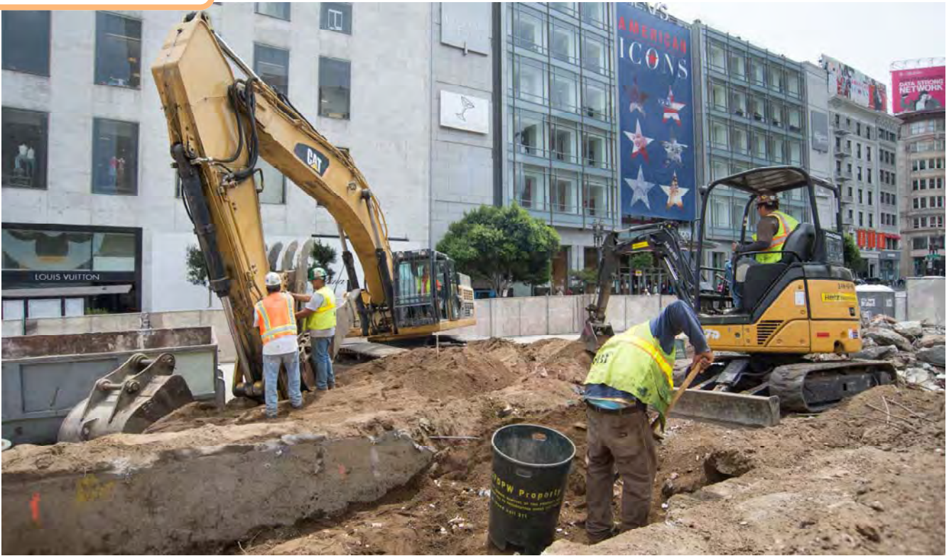
Soil is sifted and sorted from other building materials before being removed offsite.
