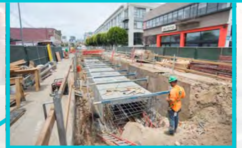
4th St. Surface Track, Systems (STS)
