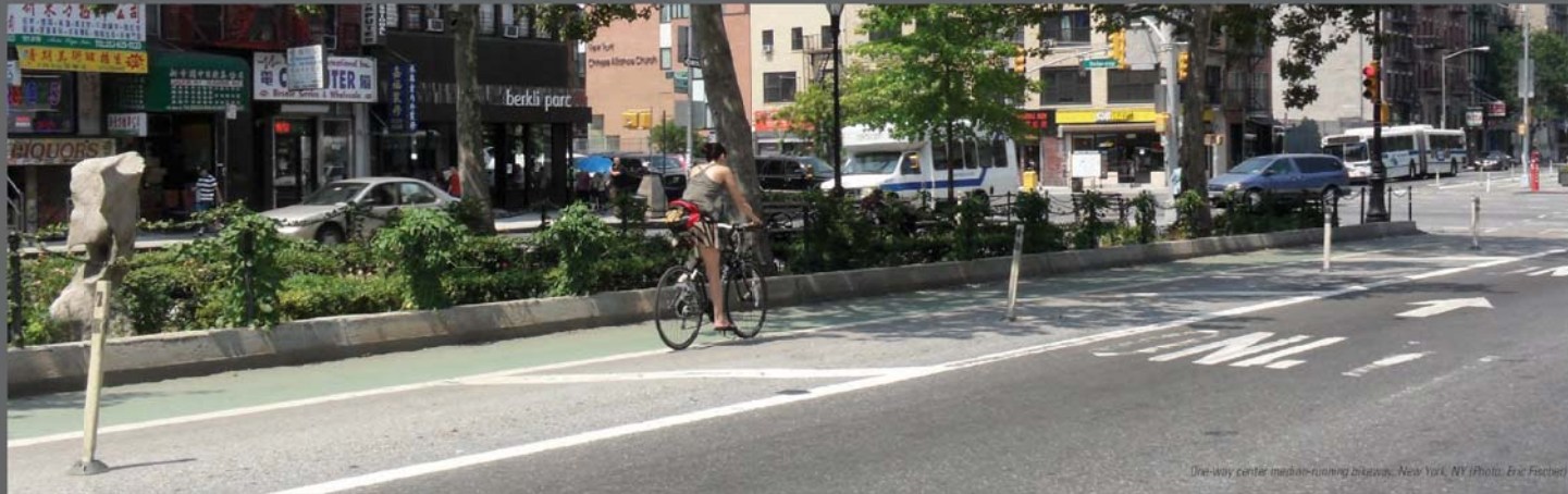
One-way center median-running bikeway, New York, NY (Photo: Eric Fischer)
