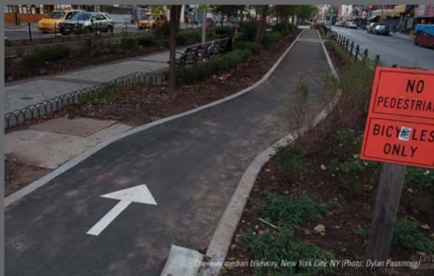
Center median bikeway, New York City, NY (Photo: Dylan Passmore)
