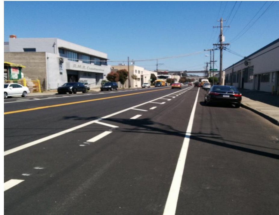
Buffered bike lane with repaving along Oakdale
