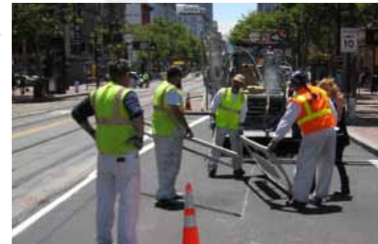
Sustainable Streets Paint Crew installing sharrows on a newly-paved Market Street.
