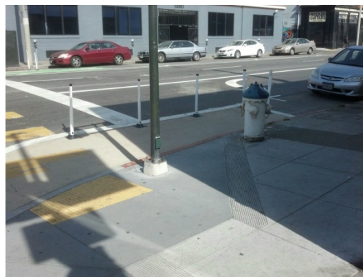
Image 3: Example of Painted Safety Zone
