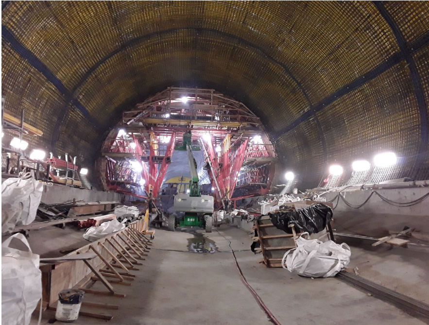
Reinforcing Mat Installation
