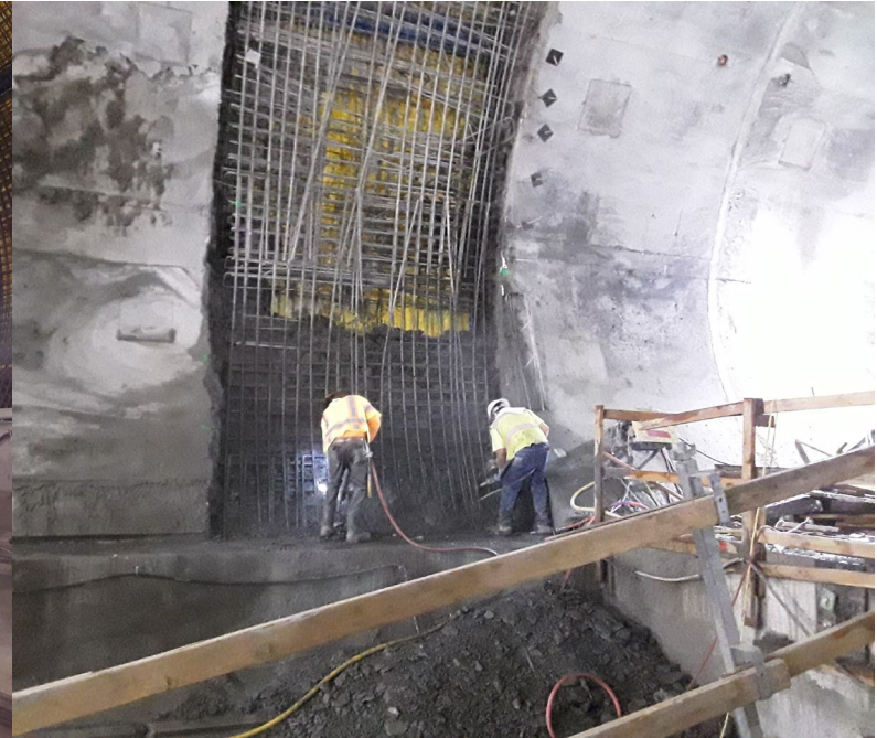
Cleaning Concrete in Preparation for Next Pour
