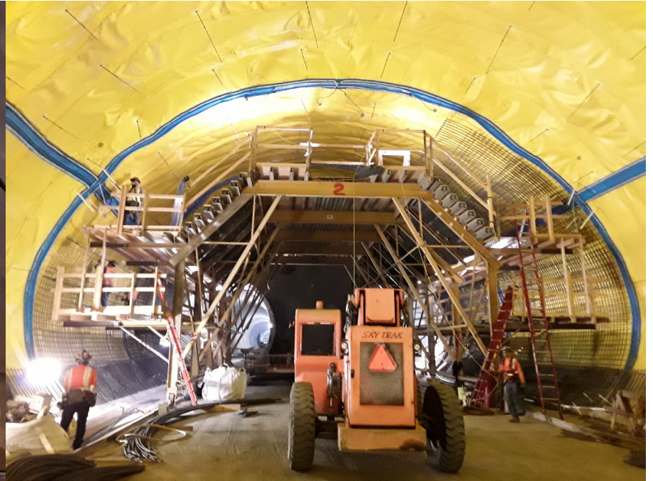
Reinforcement Rebar Installation
