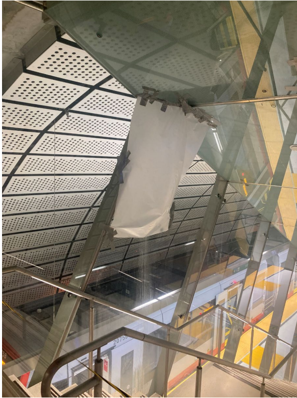
Water On Staircase
