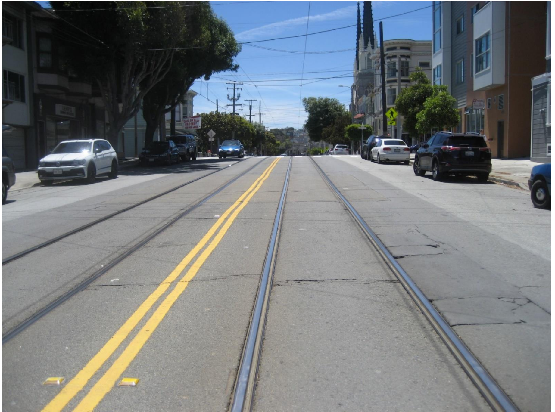
Church St, approaching 28 th St – looking south
