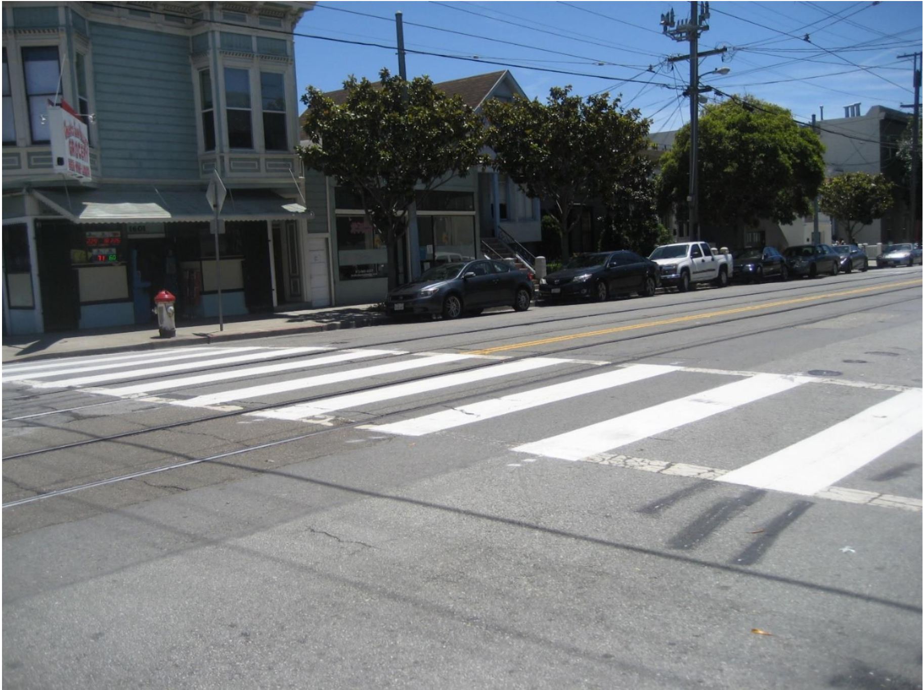
28 th St, approaching Church St - looking south (inching forward)
