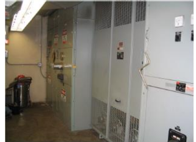
Medium Voltage Service Entrance Switchgear, 2.5 MW Medium Voltage Transformer and 480 V Switchboard
