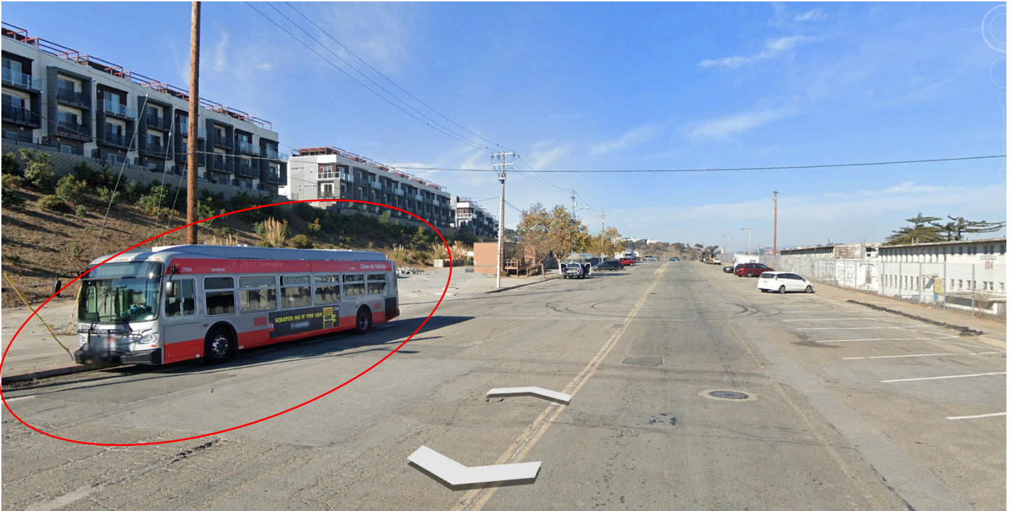
Streetview of Existing Galvez Terminal (looking north)
