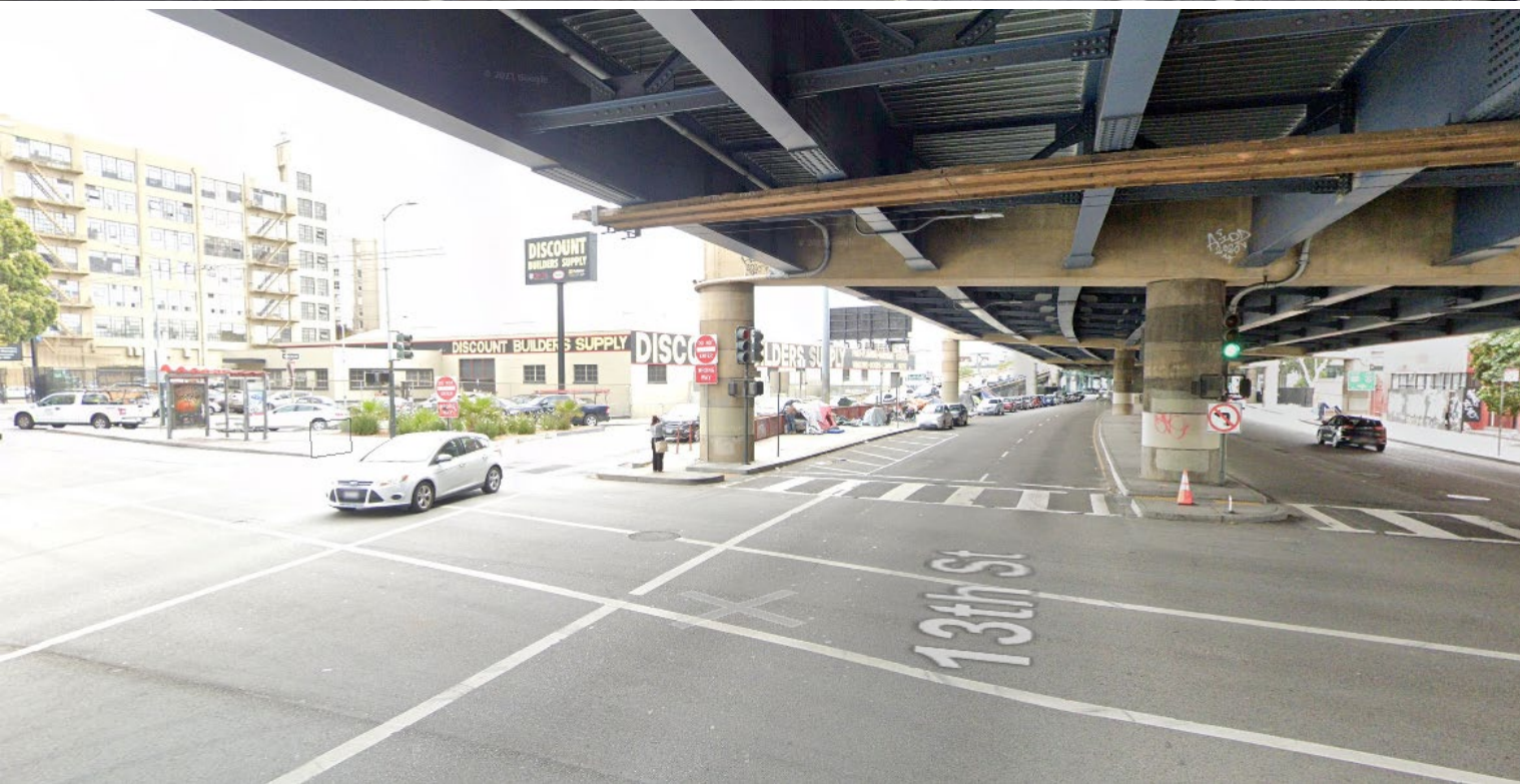
13 th Street at Mission Street/101 Off-Ramp, facing northeast
