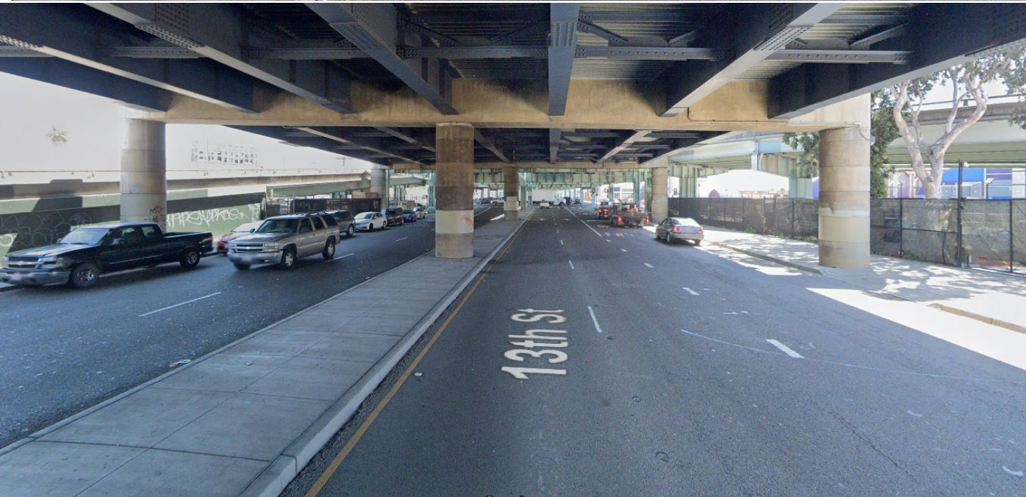
13 th Street between Otis Street/Mission Street and South Van Ness Avenue, facing east
