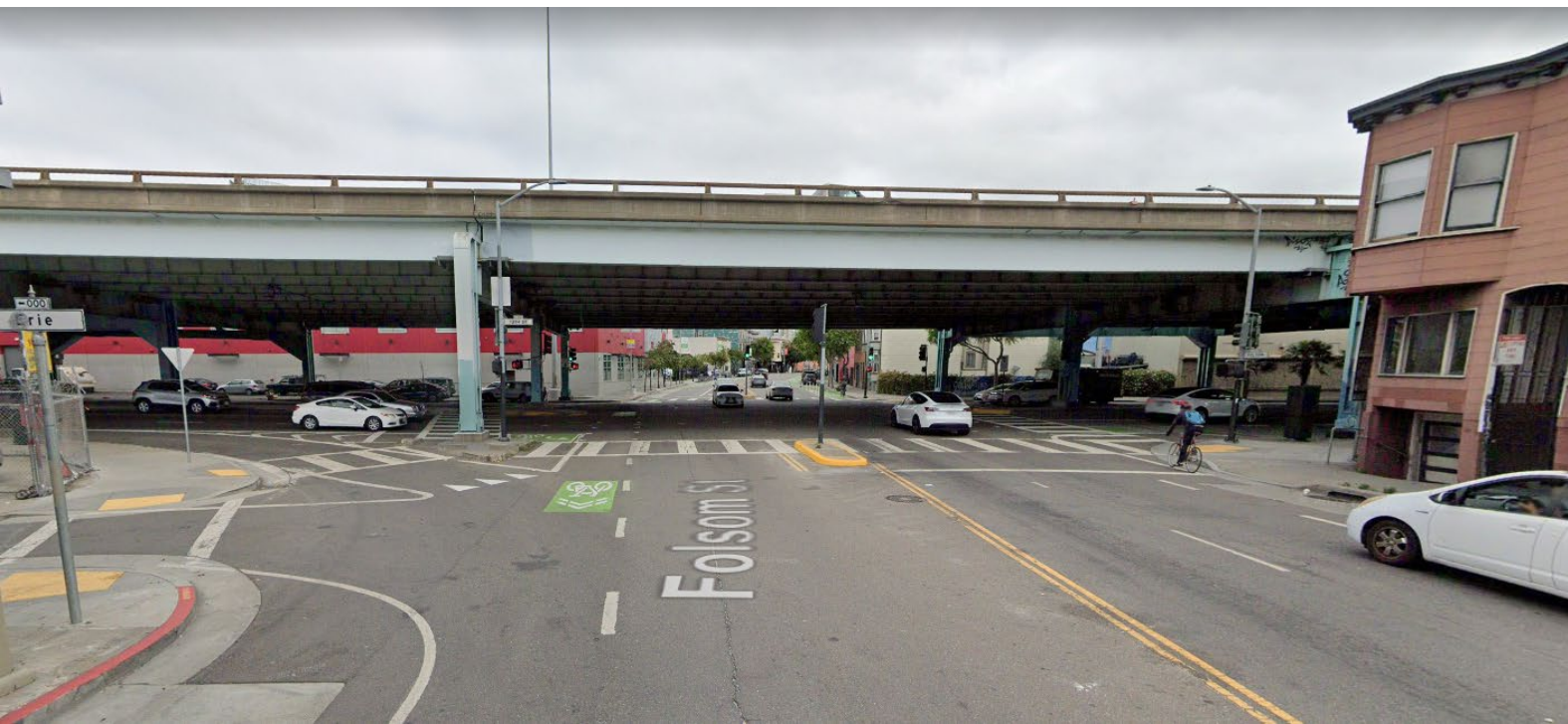
13 th Street at Folsom Street, facing north
