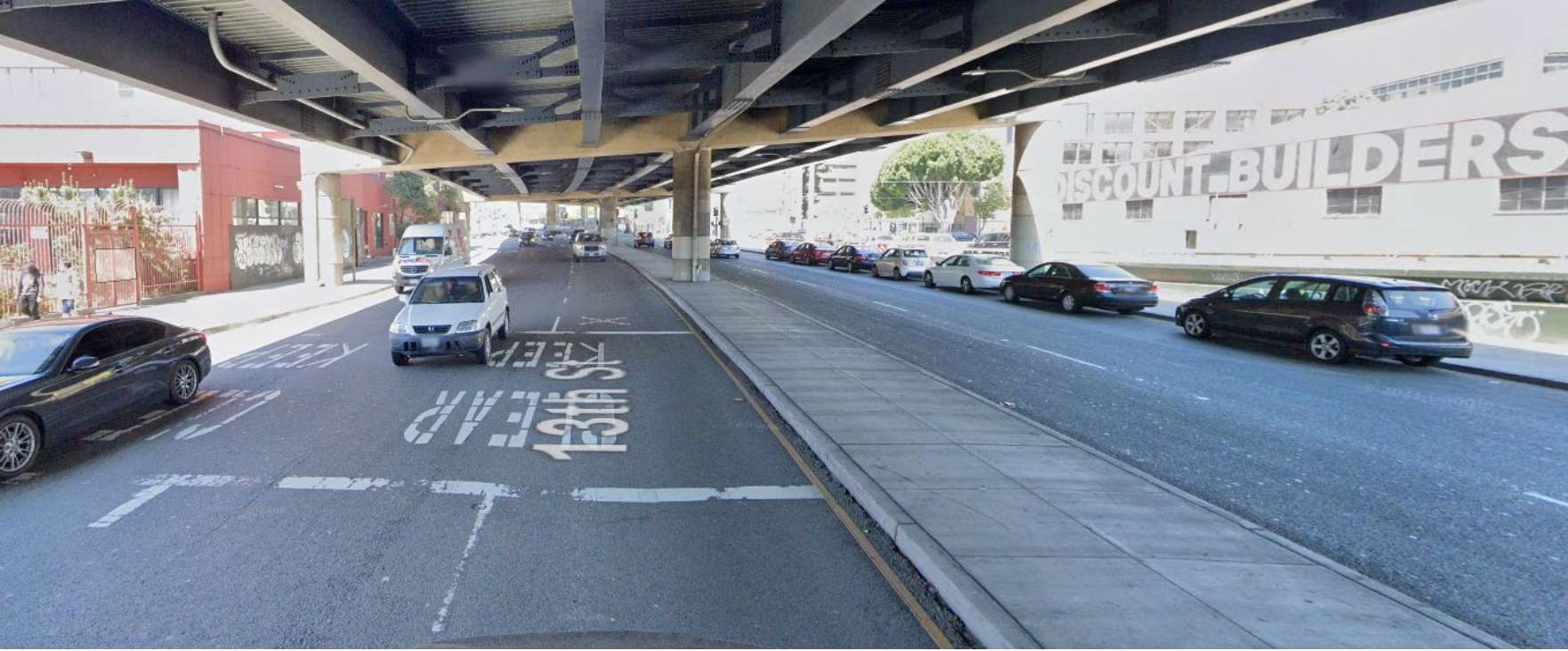
13 th Street between Otis Street/Mission Street and South Van Ness Avenue, facing west
