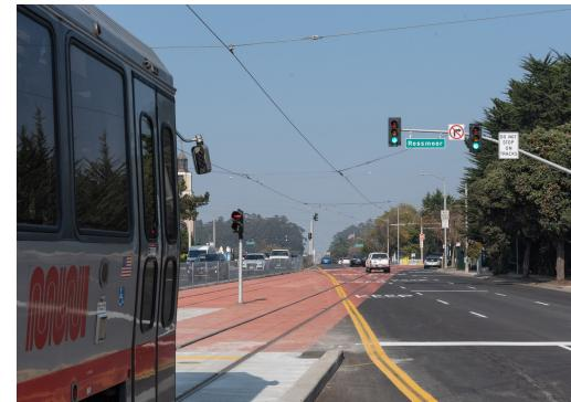
Replacing all-way stop signs with **traffic signals** can reduce transit delay. It also enables **transit signal priority (TSP) technology** at intersections that holds a green traffic signal phase as a bus approaches to reduce delays, while providing a more comfortable experience for people crossing the street.
