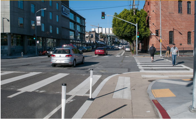
Paint, signs, and delineators
