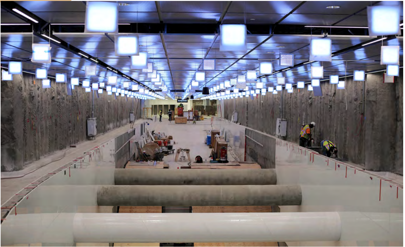
Concourse level walkway, with workers working on wiring.
