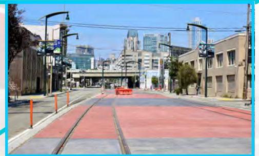
4th St. Surface Track, Systems (STS)
