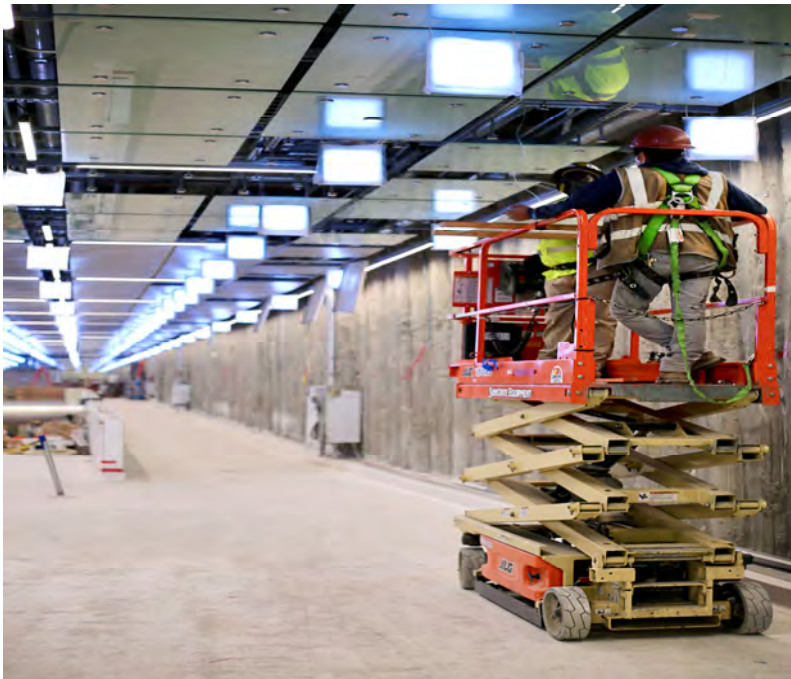
Workers using scissor lift to wire light panels
