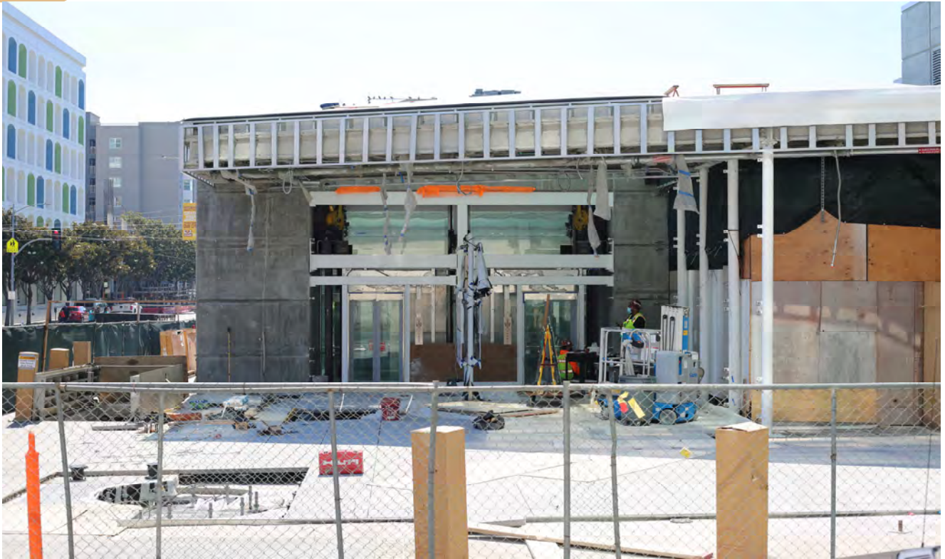
Workers working on entrance to Yerba Buena/Moscone Station surface.
