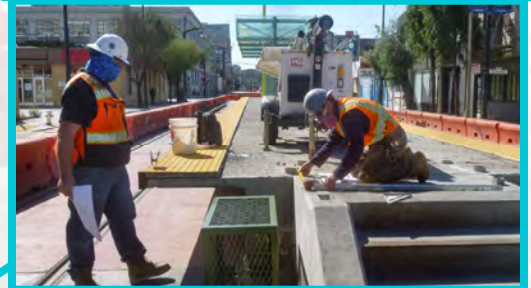
4th St. Surface Track, Systems (STS)
