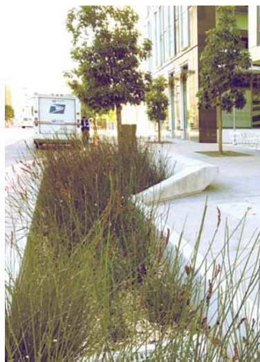
Widened Sidewalk + Stormwater Planters
