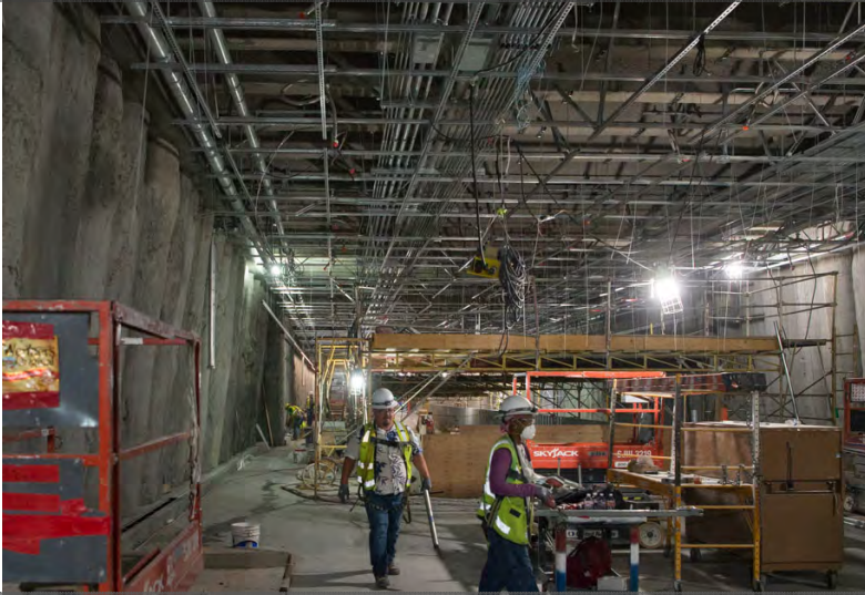
Steel framing is suspended from structural steel inside the station concourse.
