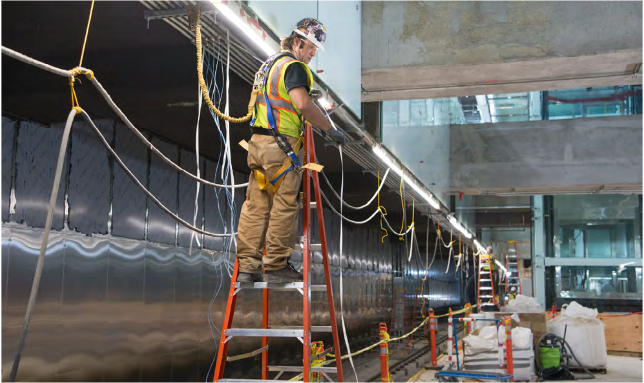
Permanent lighting is being installed on the Yerba Buena/Moscone Station platform.
