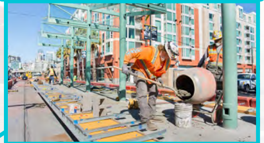
4th St. Surface Track, Systems (STS)
