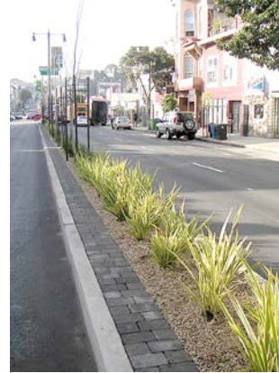
1' Maintenance Strip & Gravel Mulch
