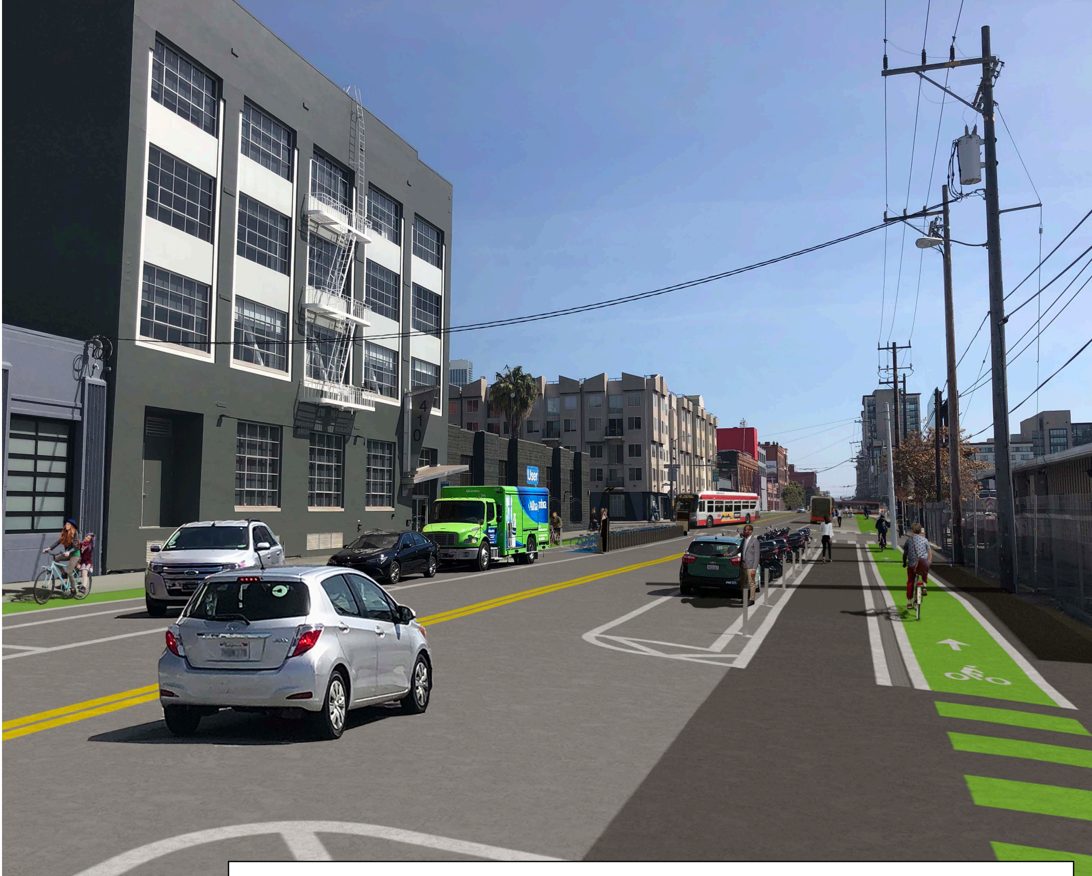
Newly paved protected bikeway and roadway-level pedestrian walkway, protected from moving traffic by parked vehicles
