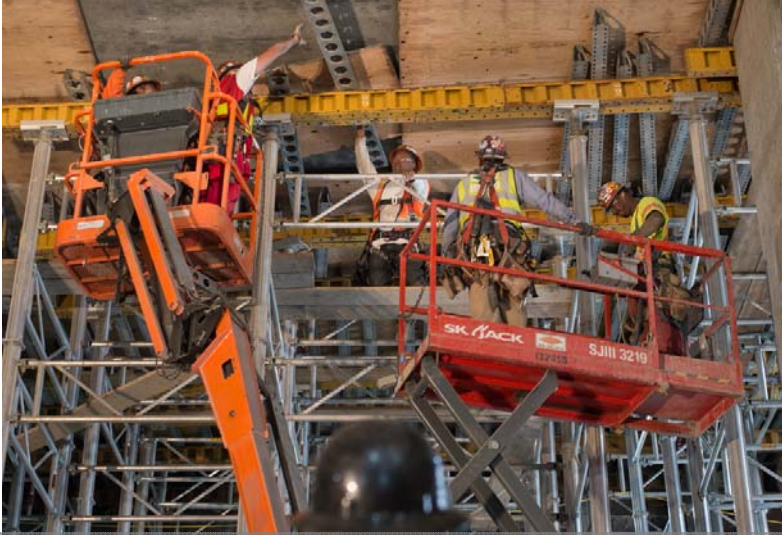
1. Adjustable struts, reinforcing, and concrete forms are placed
