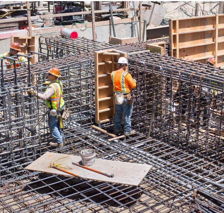
2. Rebar cages and additional formwork are installed atop bottom concrete forms
