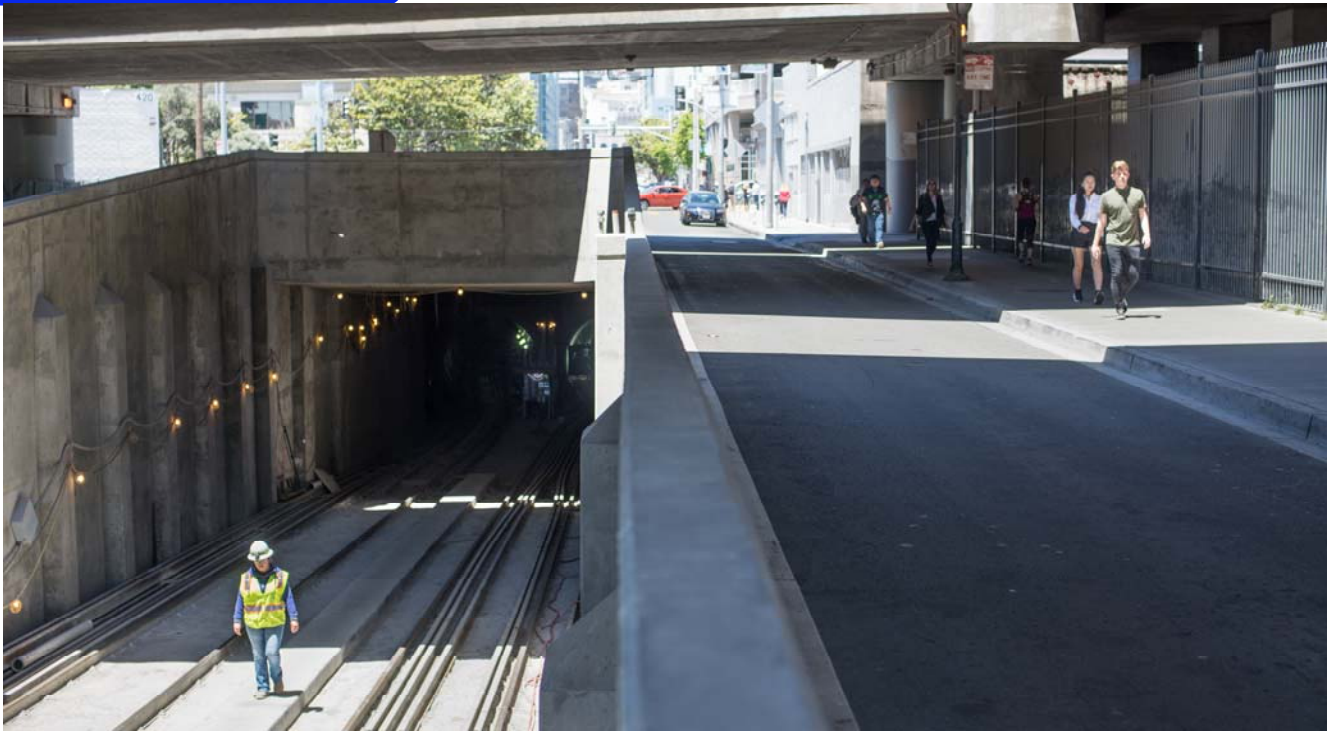
Pedestrians walk adjacent to the tunnel portal between Harrison and Bryant, as a worker simultaneously emerges from the bottom of the portal ramp.
