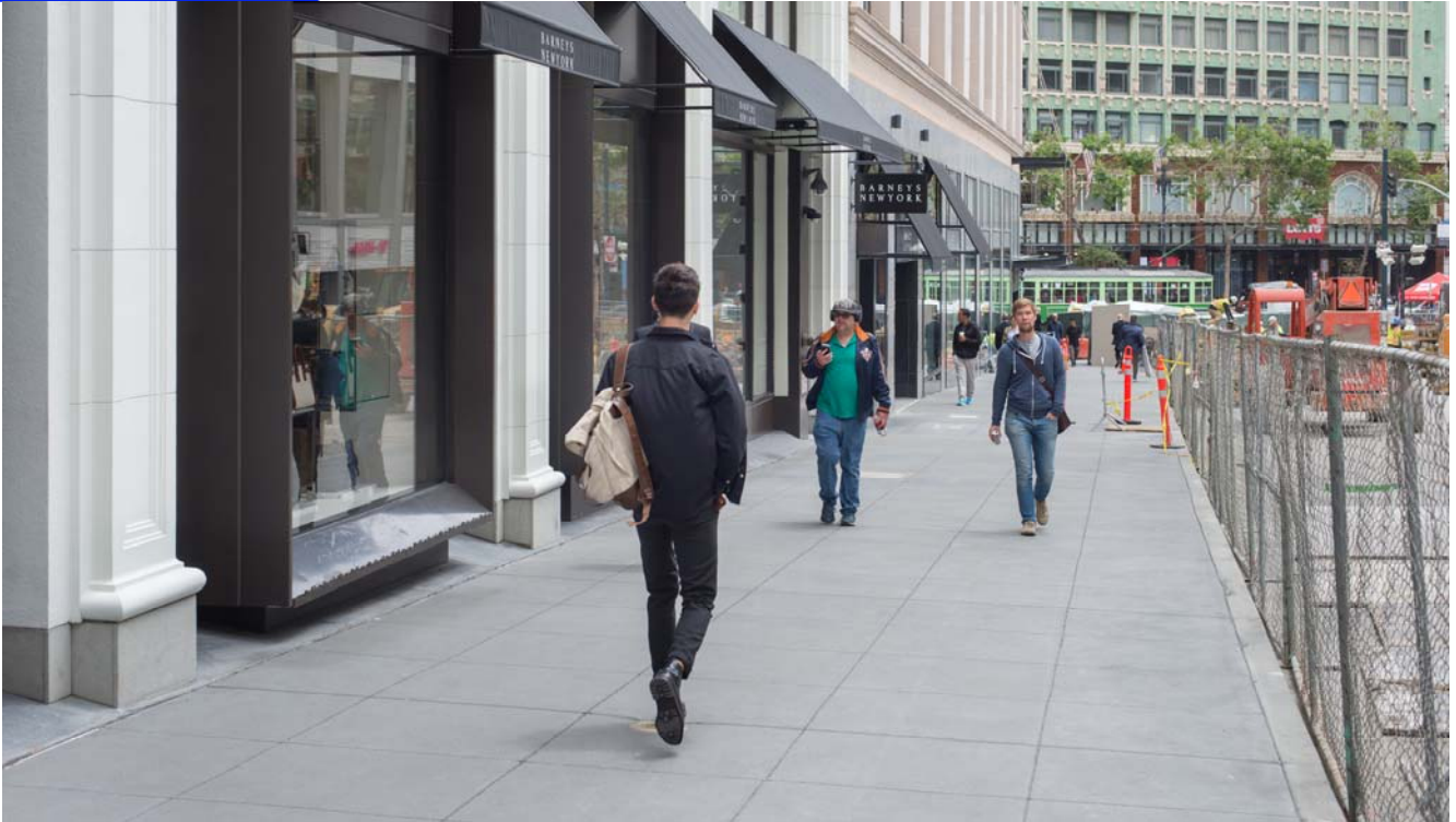
Pedestrians use the recently-restored sidewalk on the east side of Stockton between Ellis and O'Farrell.
