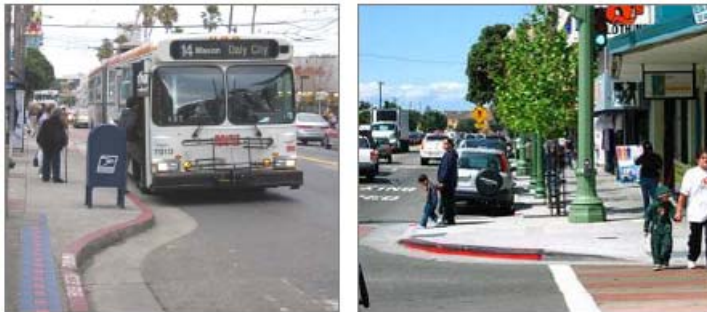
Figure 7.1 – Implementing corner curb extensions and bus bulbs on Geneva Avenue will have a benefit to pedestrian, transit passengers, and the neighborhood streetscape.
