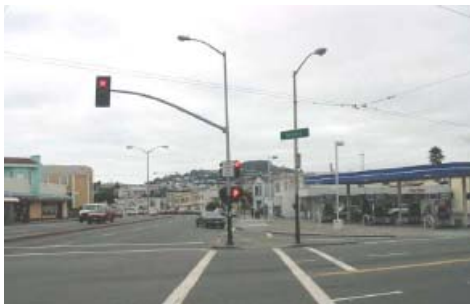
Figure 2.3 – Long pedestrian crossing distances at the Mission / Geneva intersection
