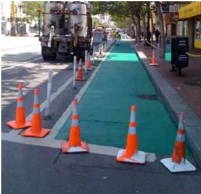
Image: installing safe-hit posts on Market Street to separate the bicycle lane from the traffic lanes
